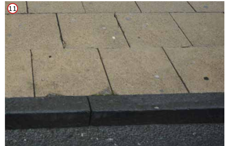
The quality of hard landscape materials along King Street is lower than those used on Wallgate. King Street is currently paved in buff concrete paving flags, with a natural stone kerb. The highway is a standard tarmac finish.
