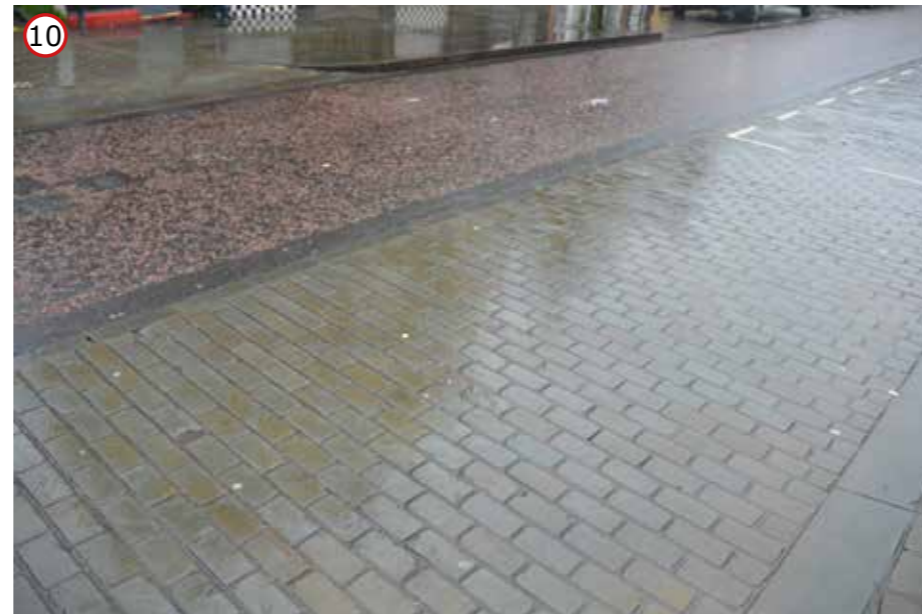
Along Wallgate high quality paving materials add to the character of the street. Sandstone setts are utilised within bus stops and loading bays. Sandstone edges define the sandstone slab footpaths and the highway is surfaced in tarmac with a red granite chipping.
