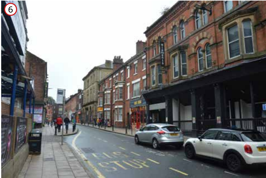
The existing arrangement of bus stop and disabled access parking bays creates a pinch point within the highway. The bus stop does however generate pedestrian movement along King Street.
