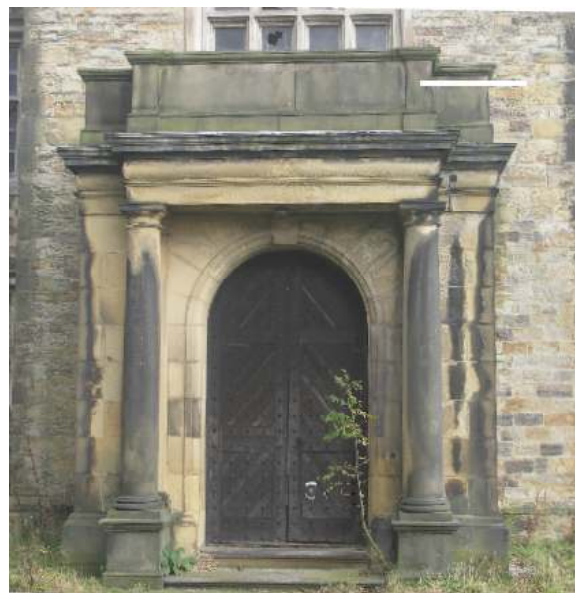
Doric Columns at Entrance to South Facade
