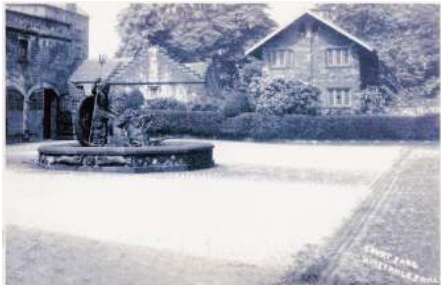
The Upper Courtyard c1900, Showing the Neptune Fountain, Estate Office and Malt House
