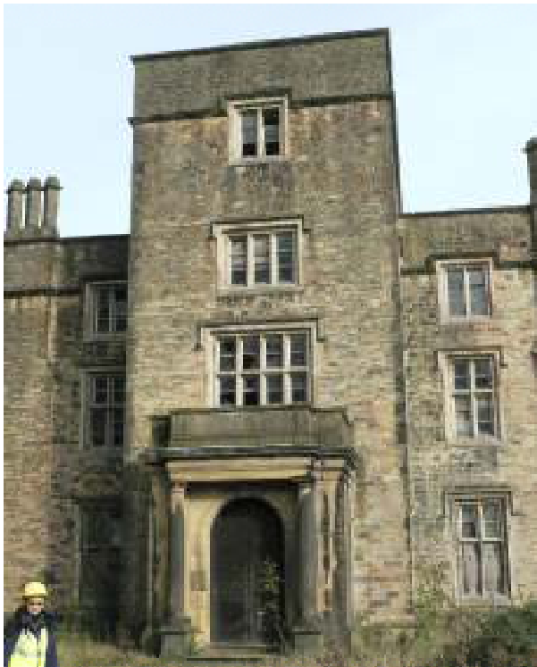
Wyatt Tower South-west Facade
