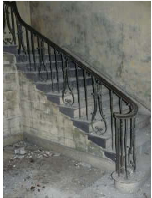
The Wyatt Staircase
