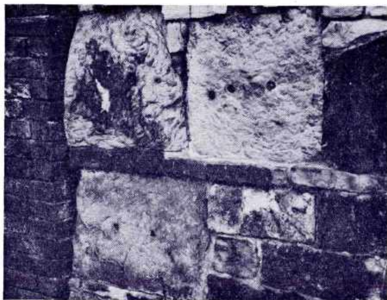
Plate 15. Stone railway sleepers built into a barn wall near No. 3 Pit.
