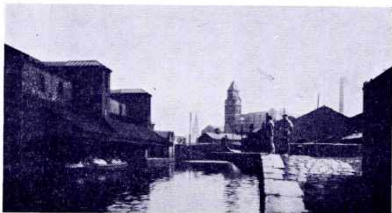
Plate 14. THE END OF THE LINE The canal waterfront at Wigan.
