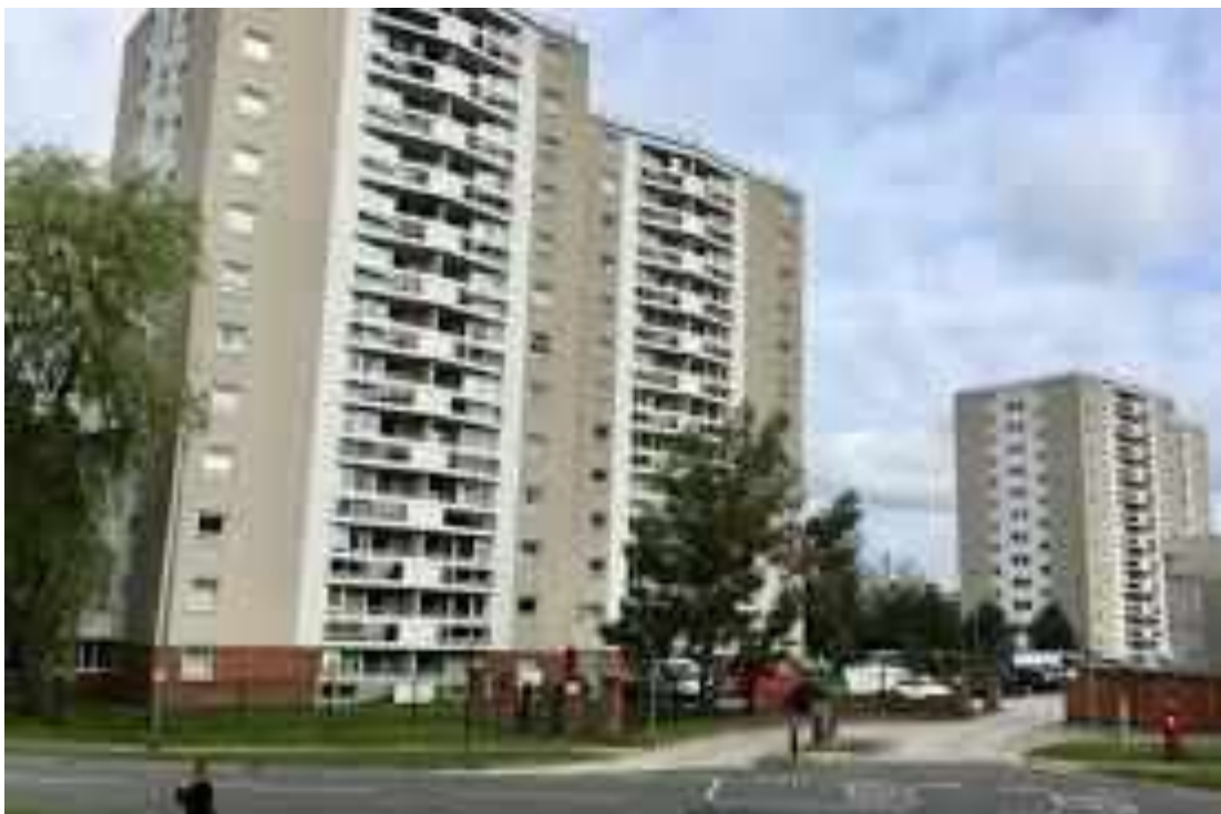
High Rise Flats Scholes, Wigan 2017
