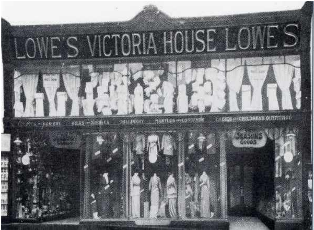
Lowe's Department Store, Market Street, Wigan
