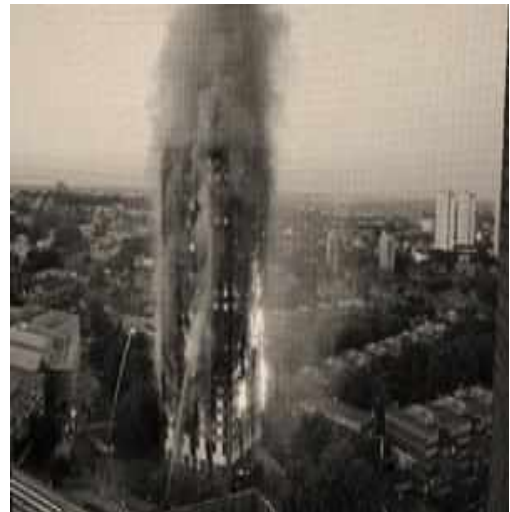
Grenfell tower fire
