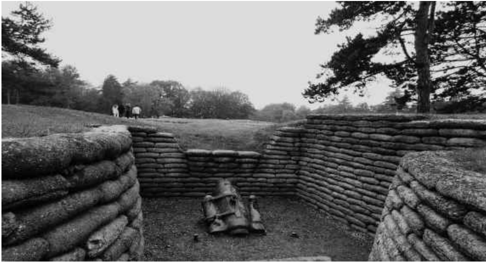
This is a reconstructed Allied trench at Vimy Ridge, Somme battlefield, showing how near the German trenches were. (Just where the group of people are standing)
