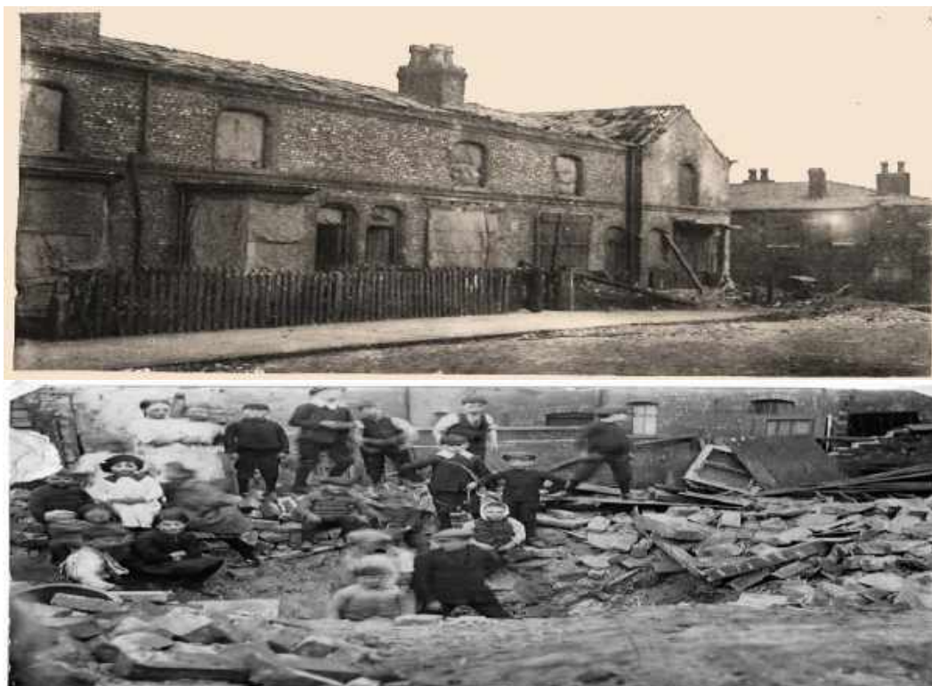
Bomb Damage, Cecil Street, Scholes, Wigan
