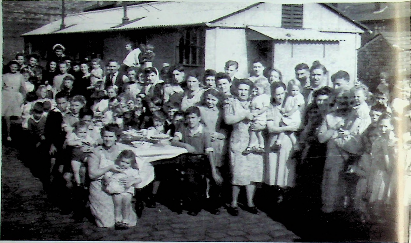
A V-E day party in St. Patrick's. The old school canteen which stood on Stewart Street is shown in the background.
