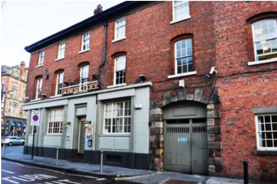
Figure 9: 2 - 6 King Street, Wigan viewed from King Street
