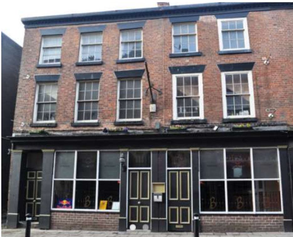
Figure 11: 7, 9 and 11 King Street, Wigan viewed from King Street
