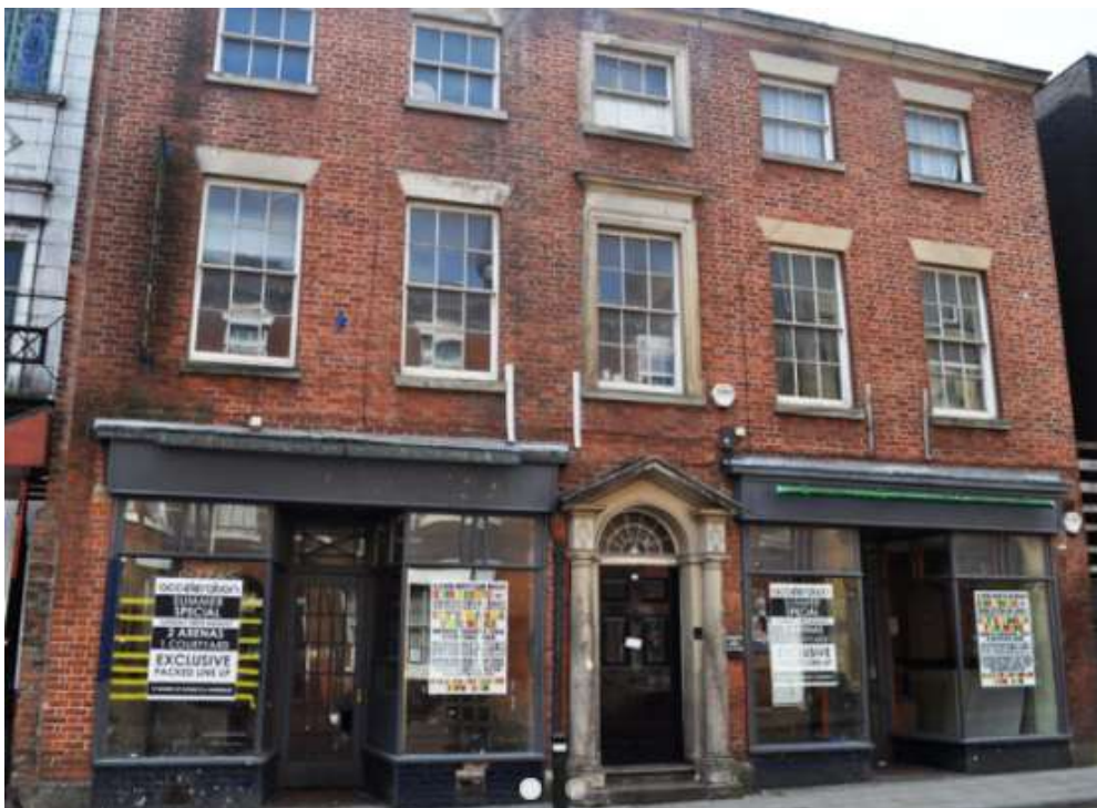
Figure 13: 21, 23 and 25 King Street, Wigan
