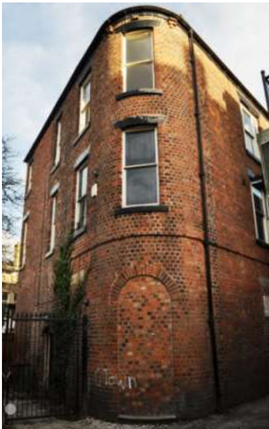
Figure 12: 13 and 15 King Street, Wigan
