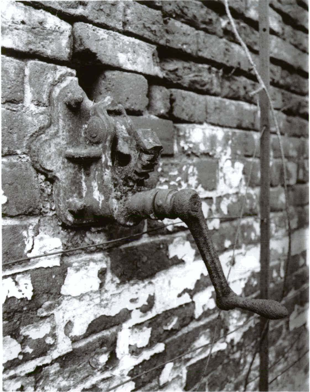
Plate 14. Glasshouse 3, worm drive for ventilation
