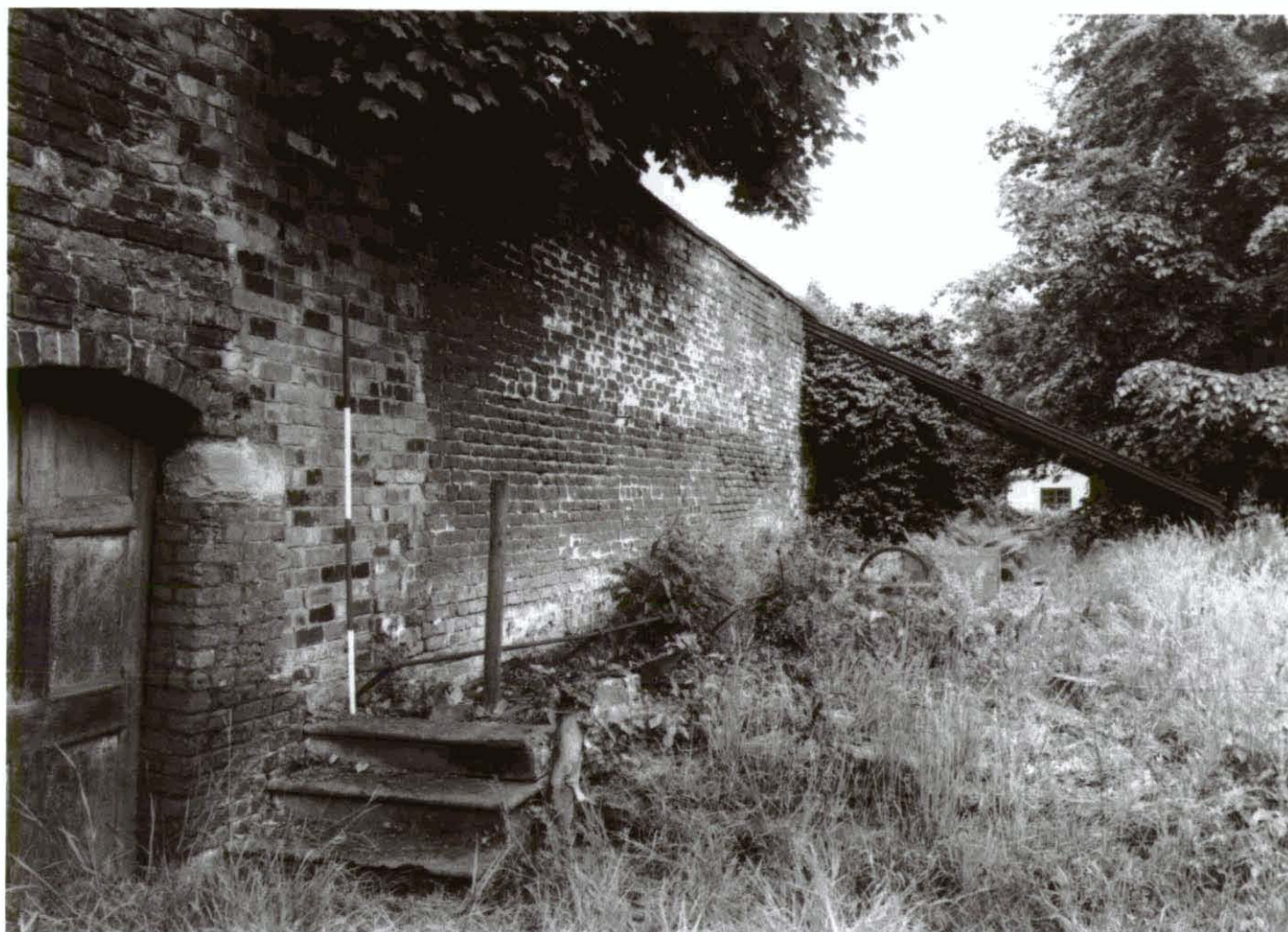
Plate 1. Glasshouses 1 & 2 from west
