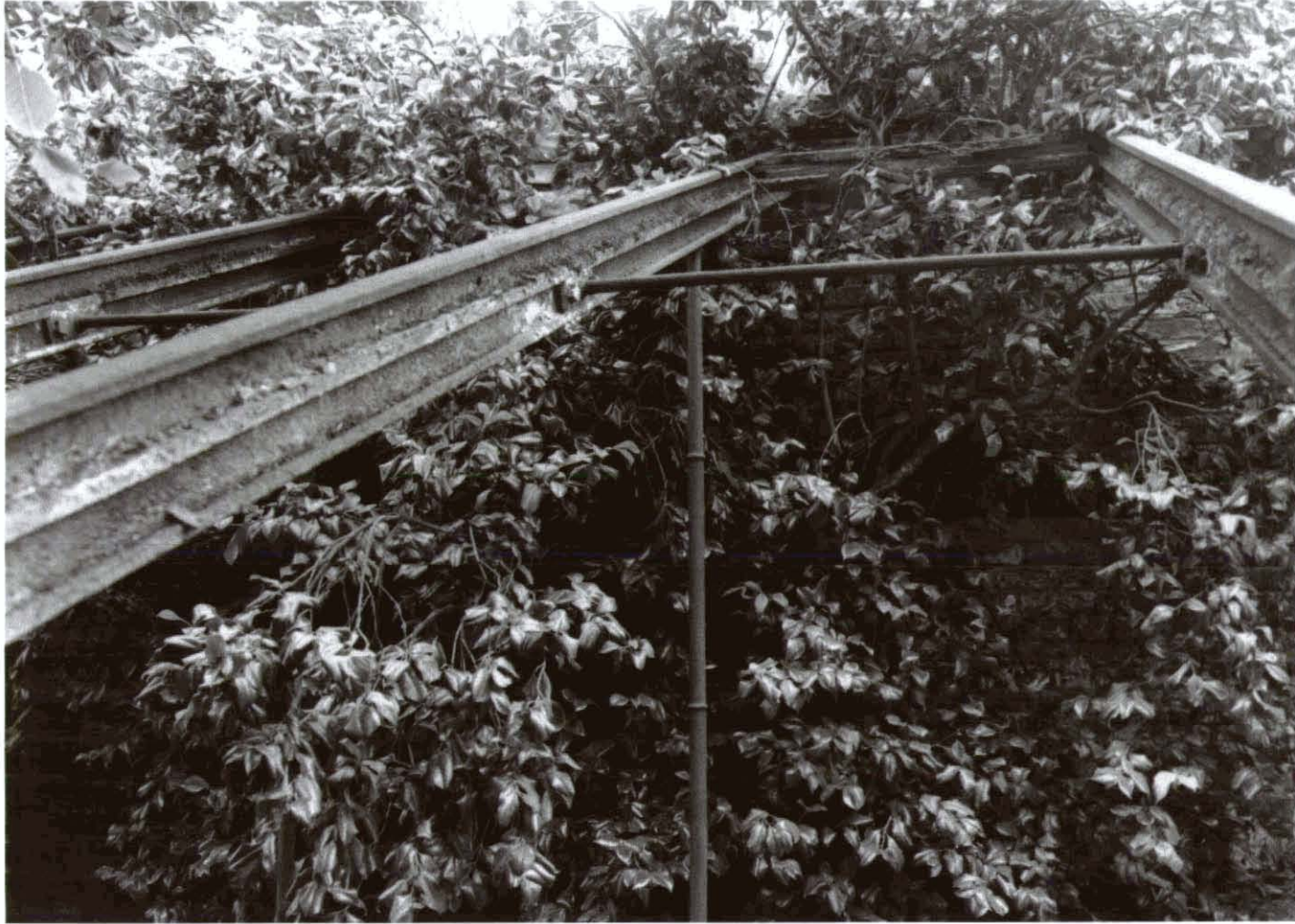
Plate 11. Glasshouse 2, roof detail from south
