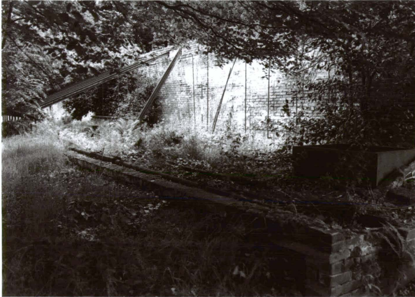
Plate 12. Glasshouse 3 from south-east
