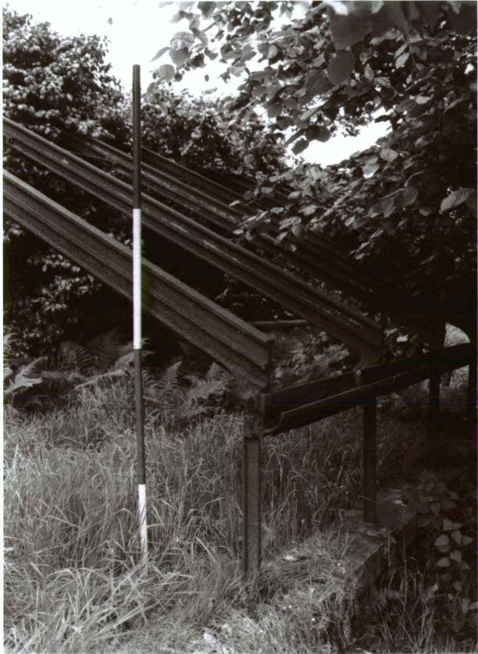
Plate 6. Glasshouse 2, from south-west
