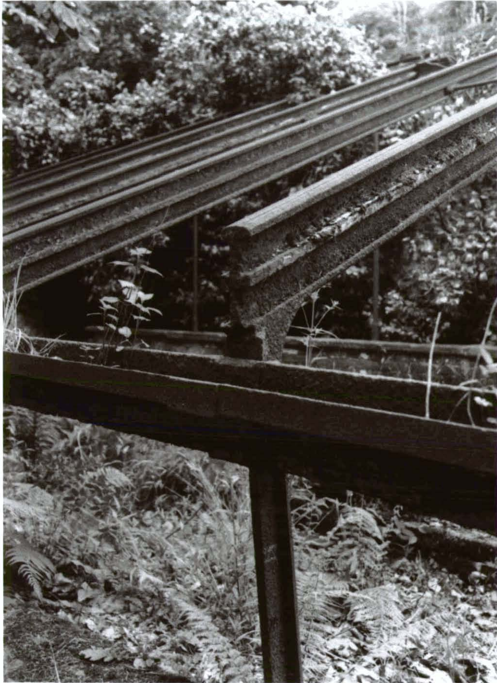
Plate 10. Glasshouse 2, cast-iron frame detail from south
