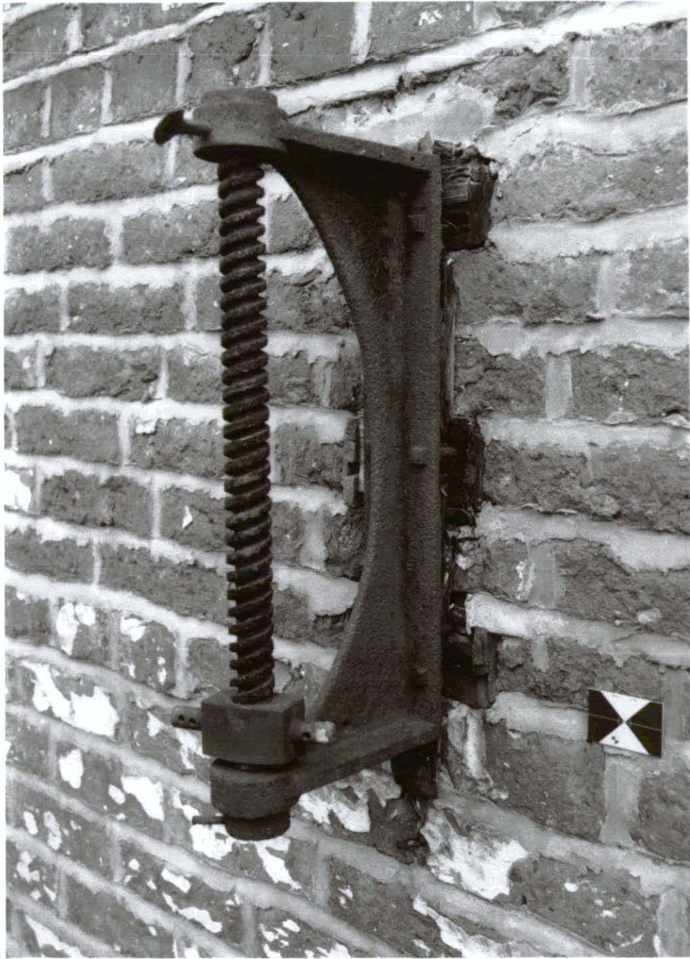
Plate 16. Glasshouse 15, worm drive for ventilation
