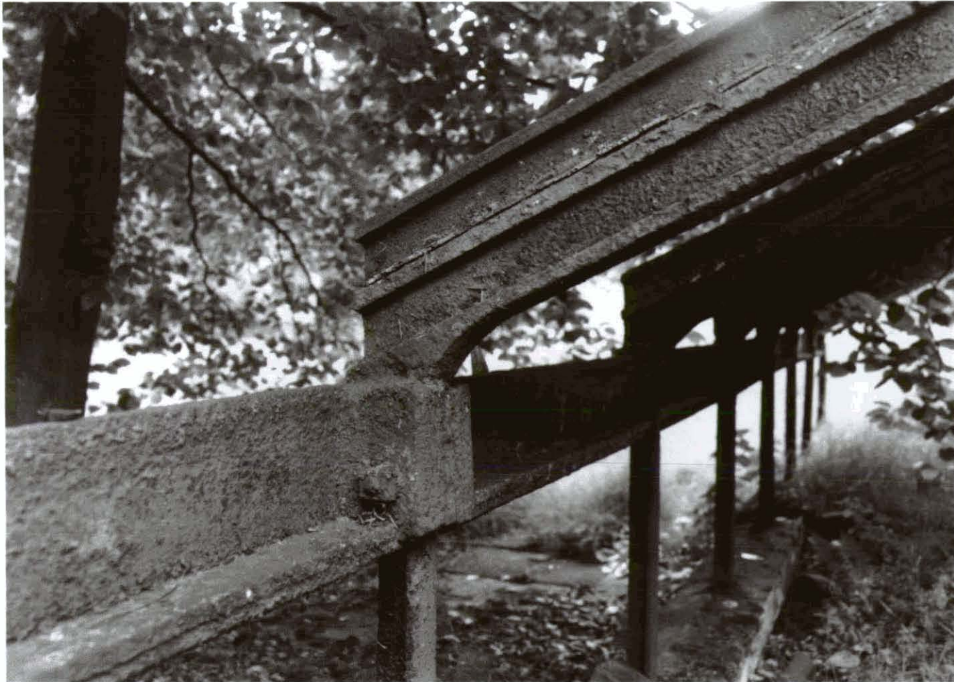
Plate 9. Glasshouse 2, cast-iron frame detail from east
