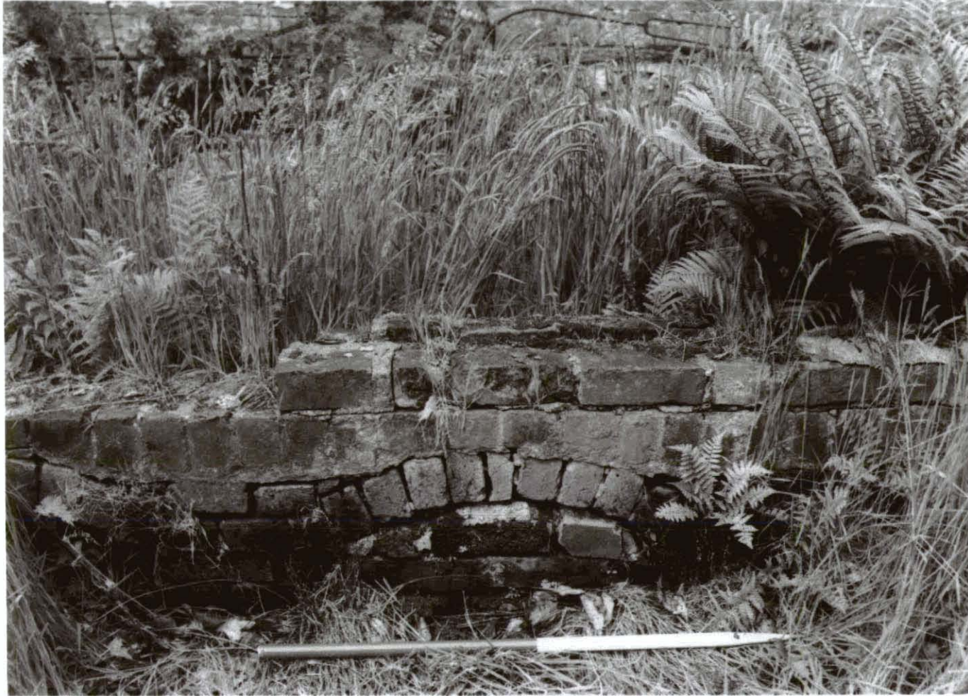
Plate 2. Glasshouse 1, vine arch from south
