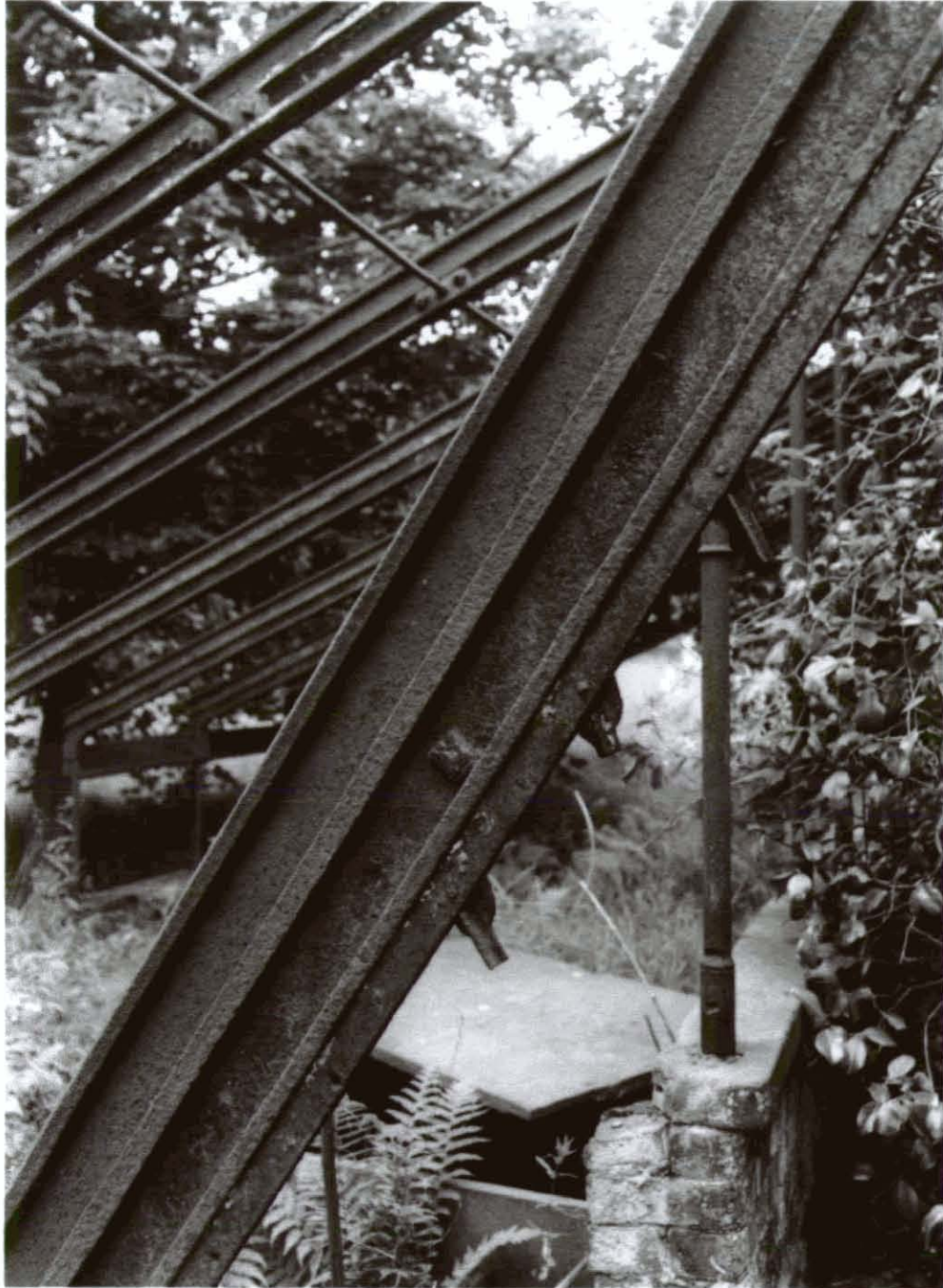
Plate 8. Glasshouse 2, cast-iron beam detail from east
