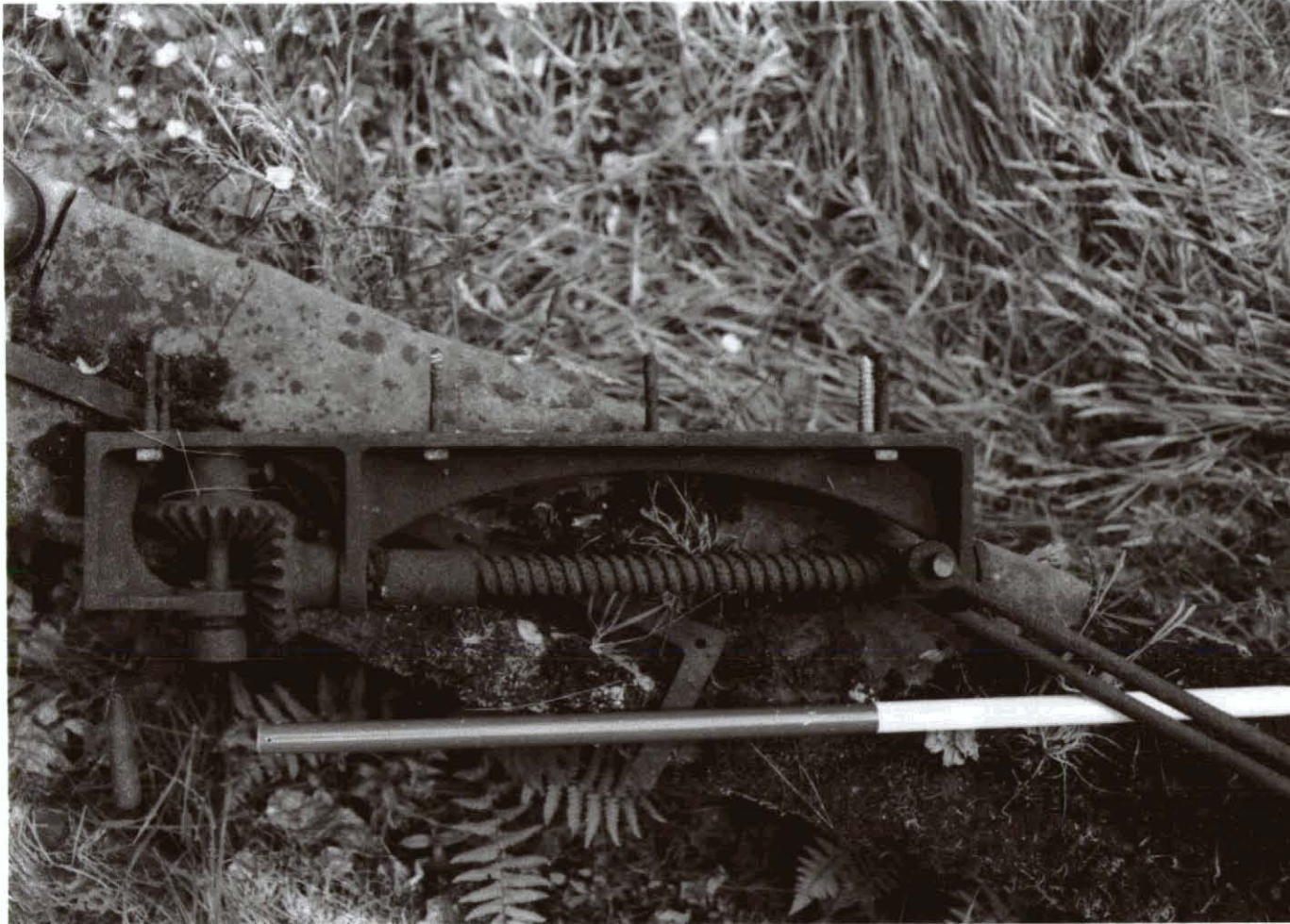
Plate 4. Glasshouse 1, displaced ventilation mechanism
