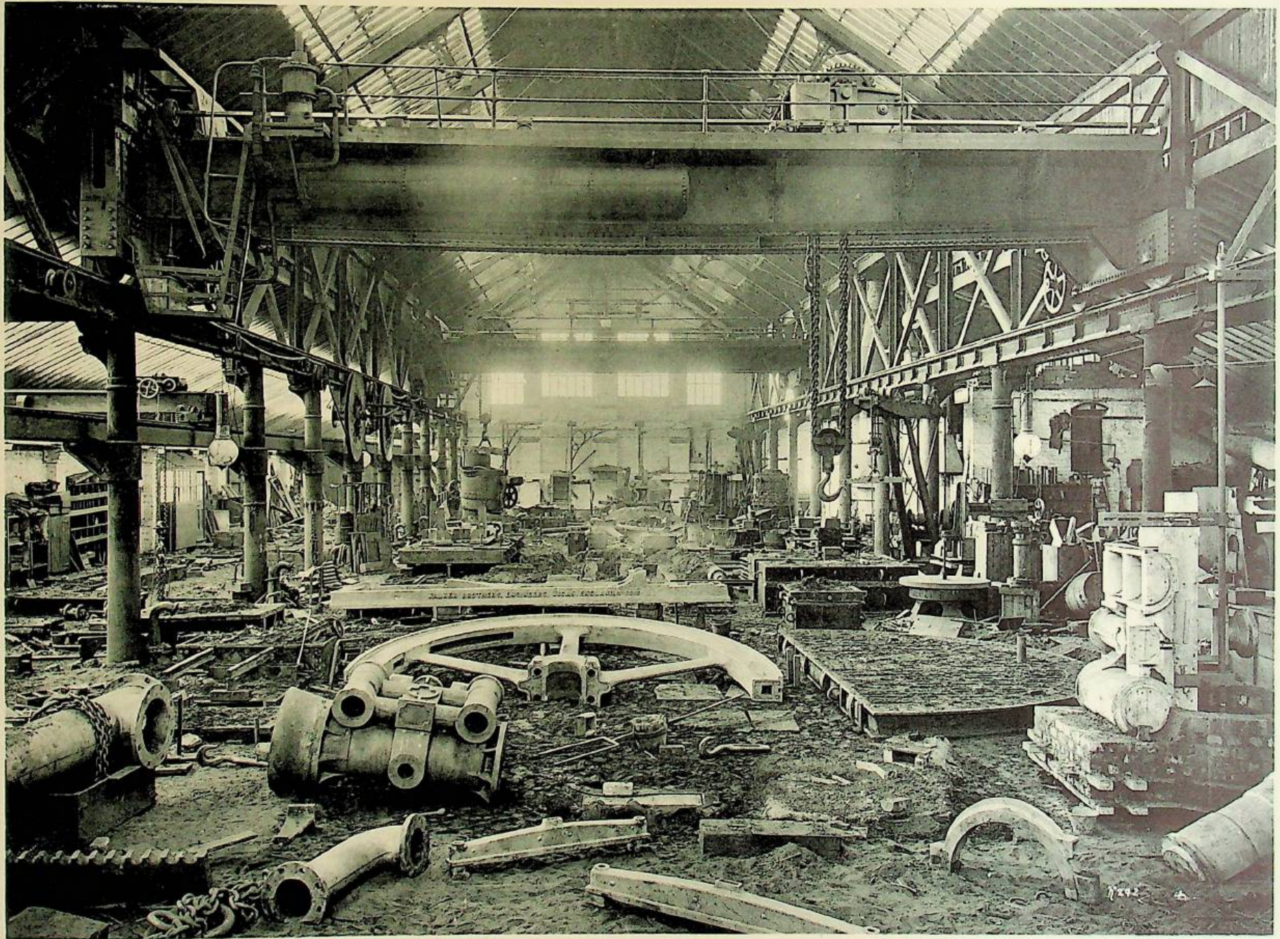
PAGEFIELD IRONWORKS.—Photo-print No. 292 shows the Interior of the Foundry at Pagefield Ironworks. The large overhead Cranes in these Works (Engine Works and Foundry) are driven by Compressed Air.
