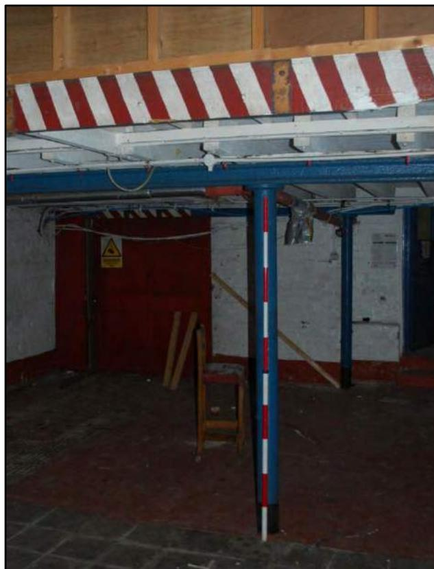
**Figure 31 Building B: secondary wall inserted across the line of window opening on ground floor. Doorway into room lined with iron plate visible.**
