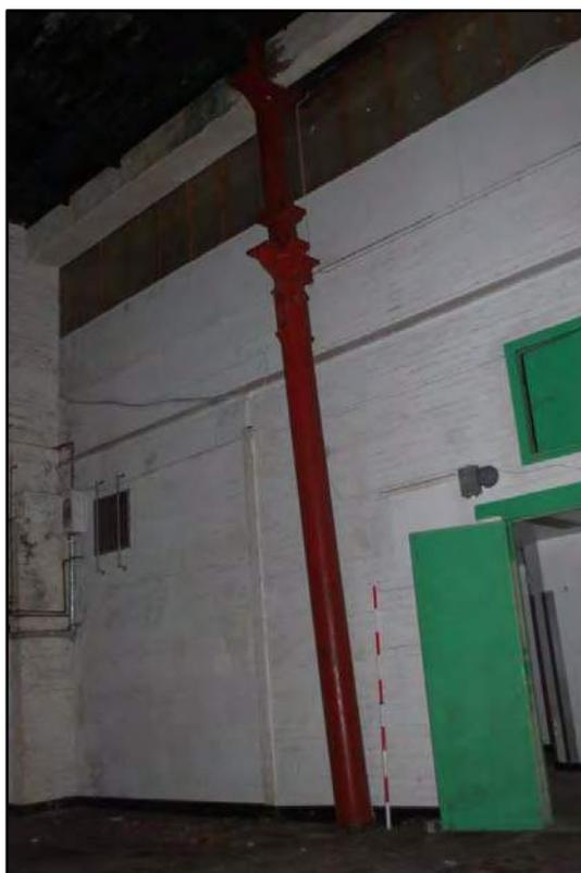
**Figure 44 Building E: detail of top of cast iron column showing housing for drive fittings**
