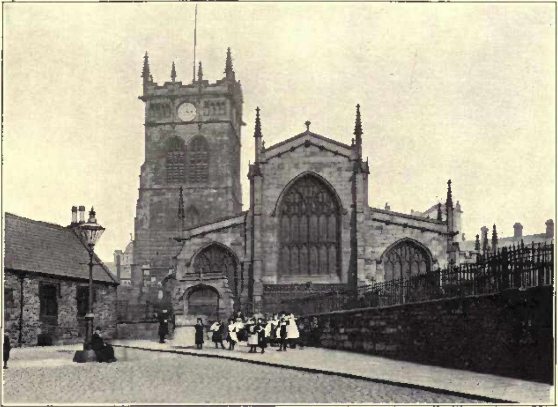
WIGAN CHURCH, FROM THE NORTH-WEST, SHOWING TOWER
