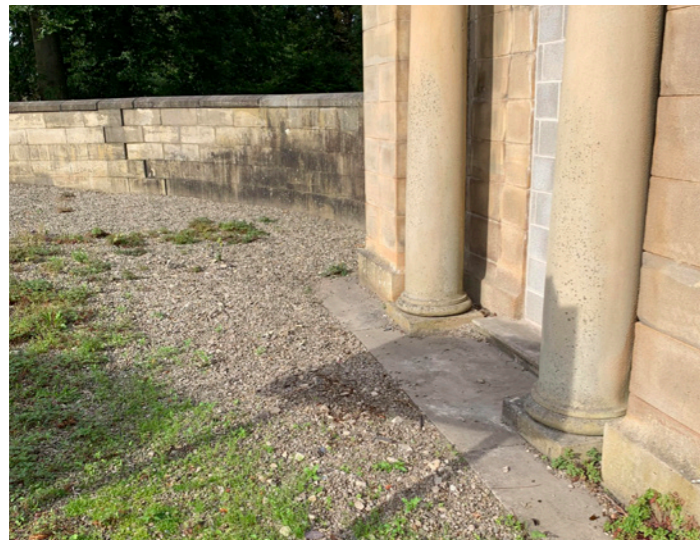
FIGURE 7.0 Showing current step access to the lodge buildings which will be replaced with level sloping access pavement.
