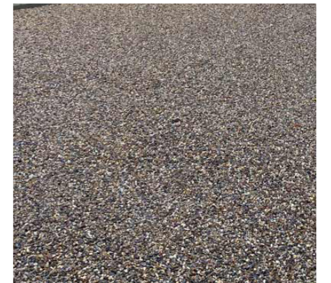
02 Pedestrian tarmac with occasional vehicle overrun
