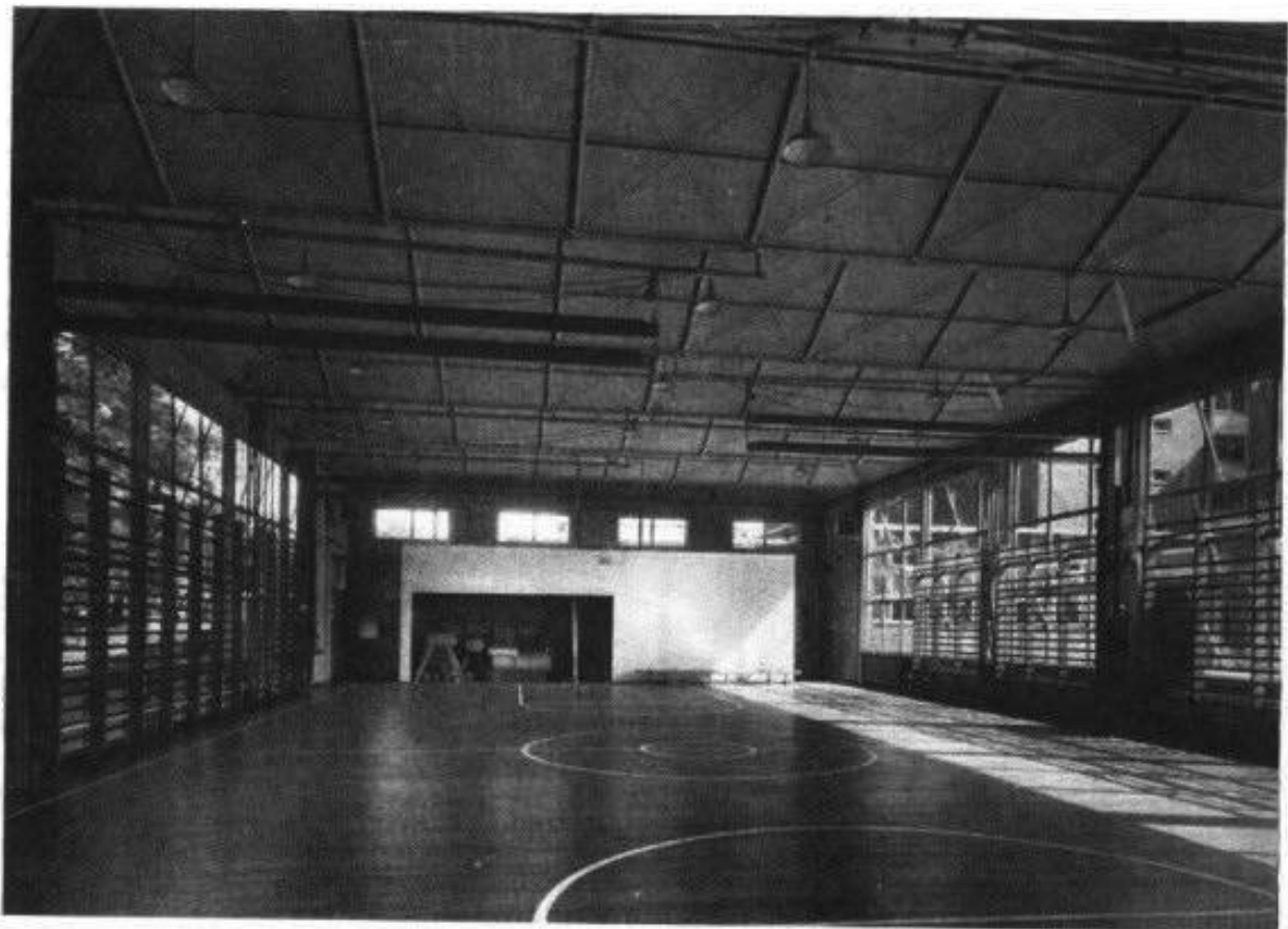
The gymnasium. The cleanness of the space frames used for the roof should be noted. Colours used have been selected to give good background for ball games.
