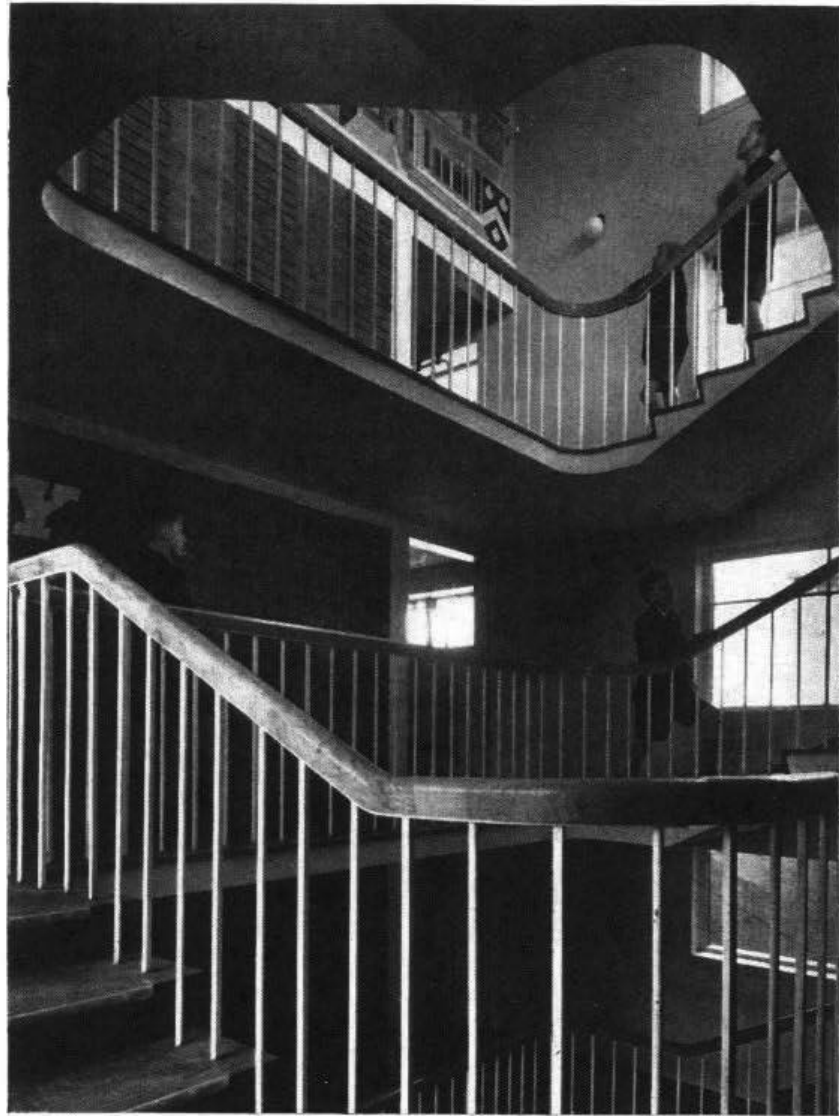
A tower staircase. The mural on the top floor is by Colin Giffard, BA, ARIBA.
