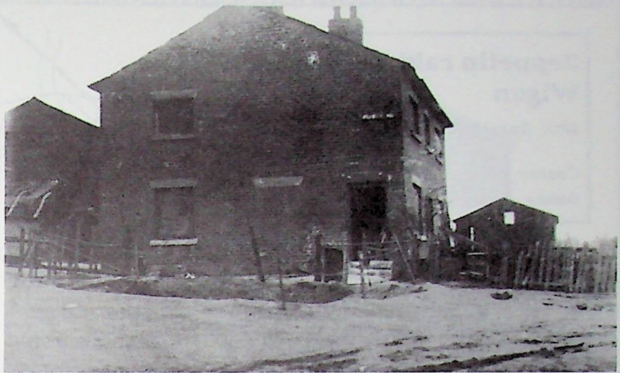
The Wigan raid. The bomb crater opposite the gable end of the house in Platt Lane
