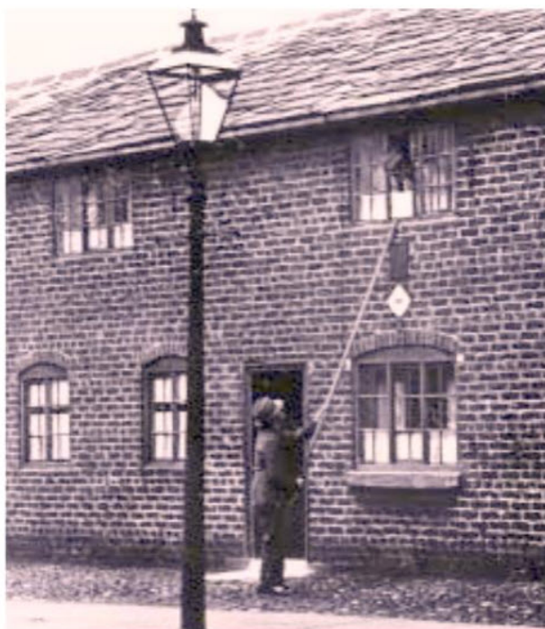
Domestic hand-loom weavers cottages formerly on Twist Lane. Note the 'Yorkshire' sash windows and knocker up.
