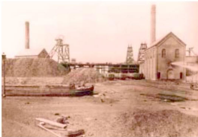
Bickershaw Colliery was developed by Ackers and Whiteley from 1872. Canal and rail links facilitated large scale mining.
