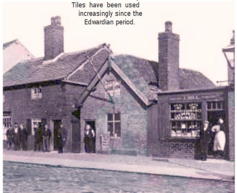
King Street roofs c.1880 ~ Thatch to the right and sandstone slate to the left. Also note the sett road surface and cobblestone inner pavement and the barber's shop pole sign.
