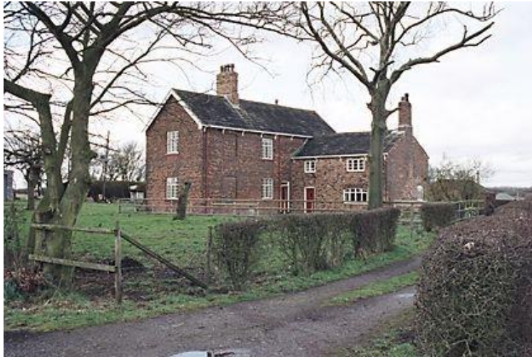
Fig. 52. Lightshaw Hall (Grade II*) at Golborne.
