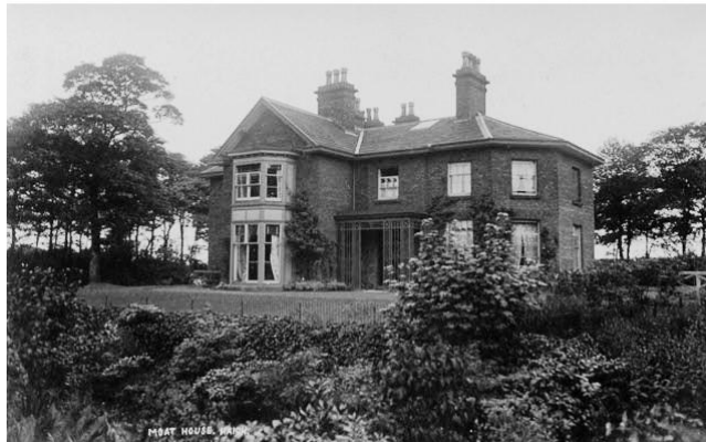
Fig. 25. Moat House (Grade II) at Haigh.
