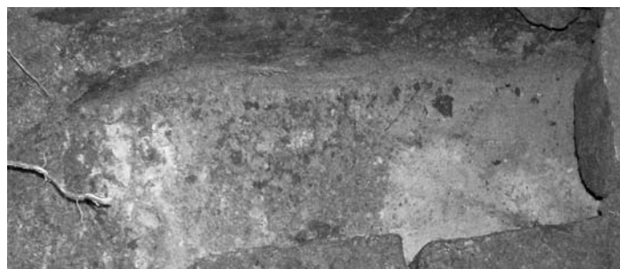
Fig 2. View showing part of the capped and un-capped suspected drain.
