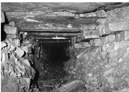
Old drainage tunnel near old pits
