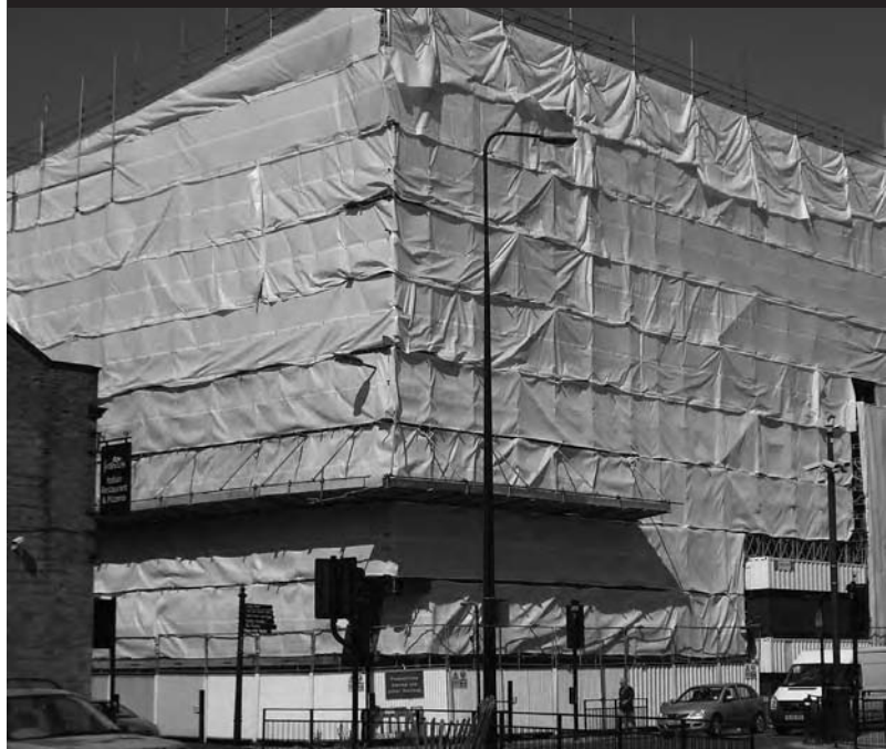
Can you see the History Shop underneath the scaffolding?
