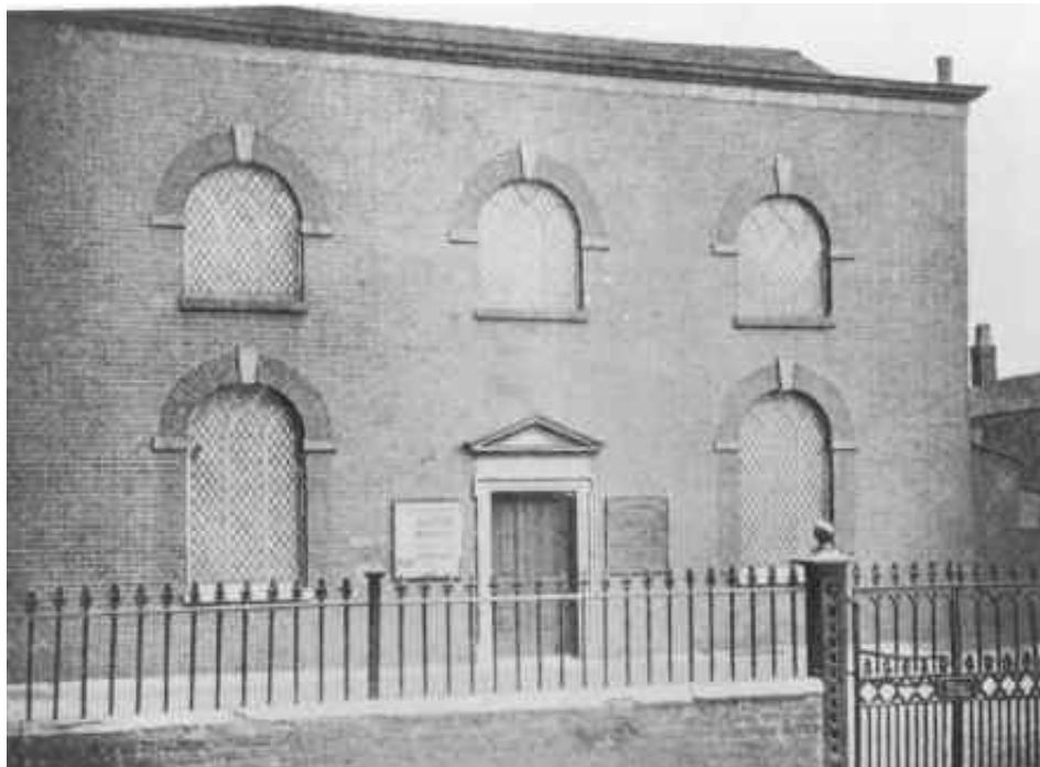
Chapel Lane, Wigan, was named after this modest building, erected in 1769
