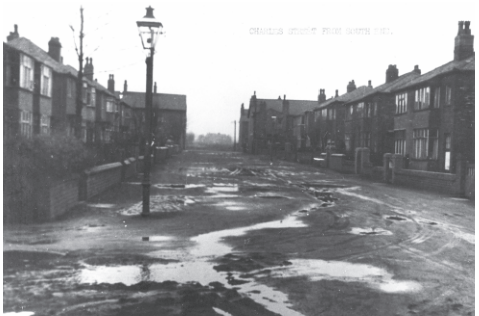
Under the Public Schemes of Work, men from Leigh were employed to pave areas such as Charles Street, Leigh
