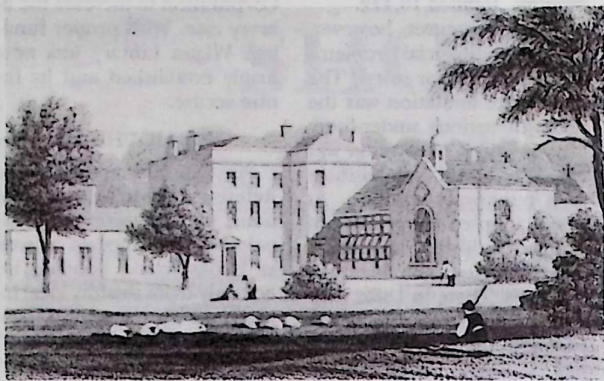
Engraving of Standish Hall, 1828. The black and white timber-framed section is the surviving part of the Tudor house, dating from 1574; the rest of the Hall was rebuilt in brick in 1748. The chapel also dates from the 1740's, while the single-storey wing was added in 1822. Most of the Hall was demolished in the 1920's.
