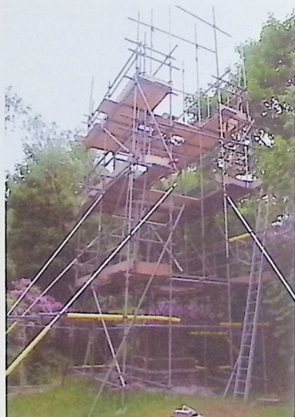
Obelisk dismantled to its plinth
