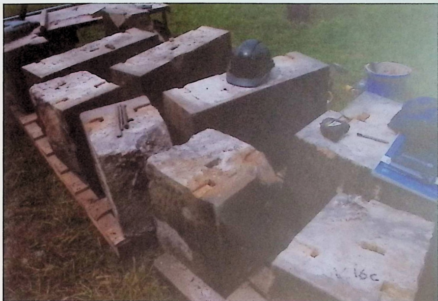
Sectional repairs
