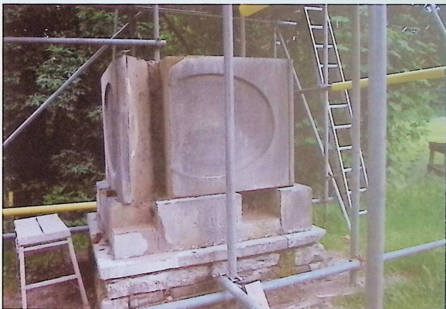
Plinth undergoing restoration work
