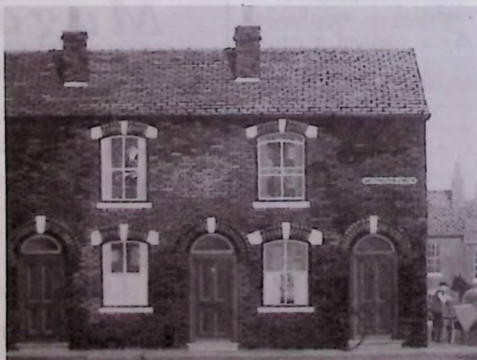
The house, no. 3 Westminster Street, Wigan (since demolished), where George Formby was born in 1904. From a painting by Gerald Rickards, based on original photographs.
