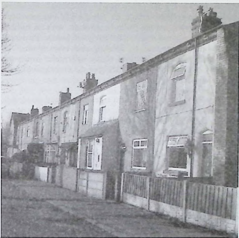
Figure 2. Miners' cottages in Victoria Terrace, Bickershaw
