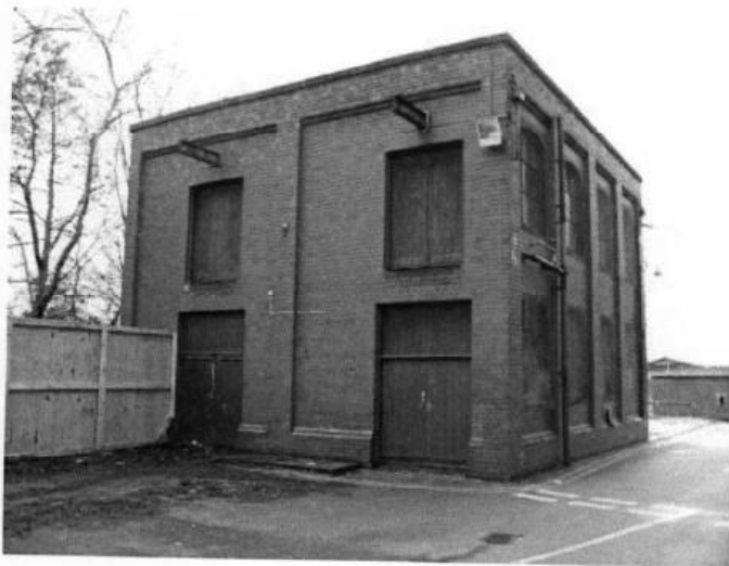
Fig.29: 1915 substation (block D)
