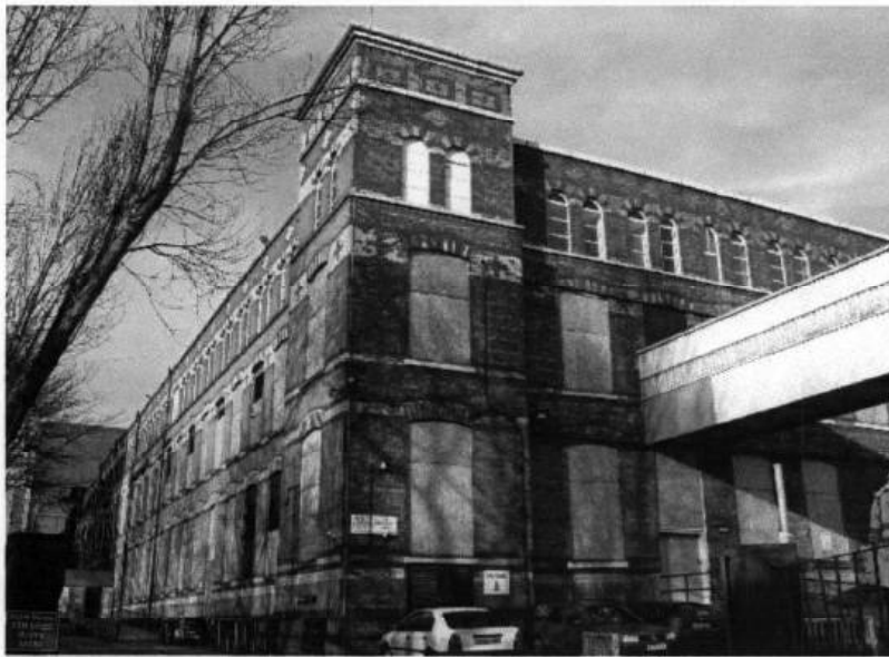
Fig. 17: south-west corner of mill and 1960s bridge
