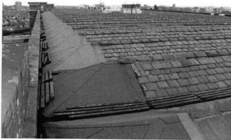
Fig.26: mill roof viewed to south-east (block B)
