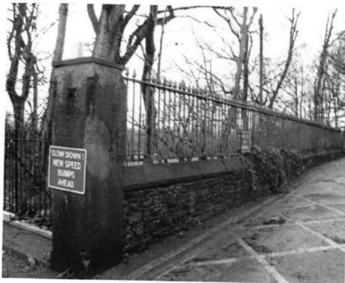
Fig.32: wall and railings along south-west boundary between Mesnes Park and mill
