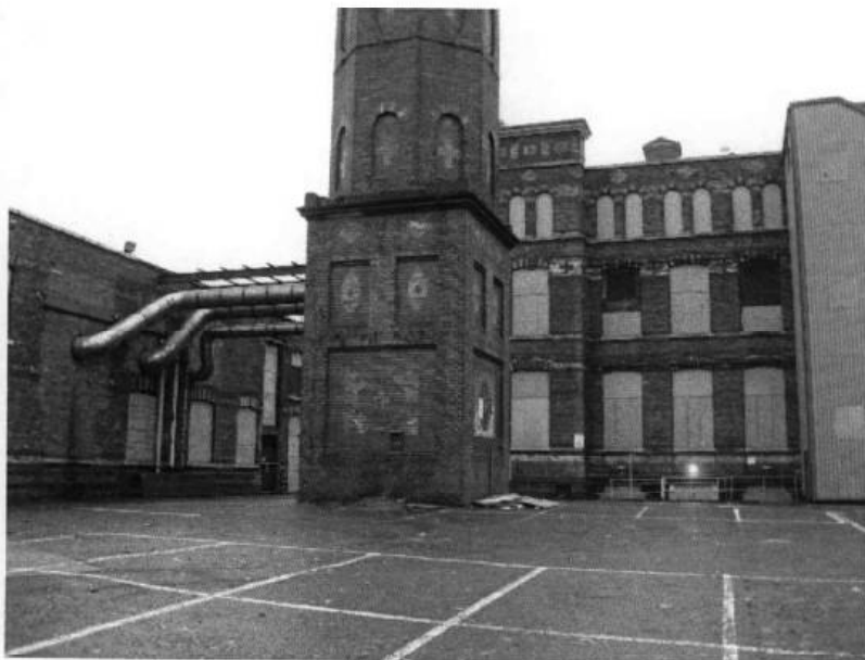
Fig.16: Part of north-west elevation of mill (block B) and chimney base, with post-war lift to right and weaving sheds (block A) to left
