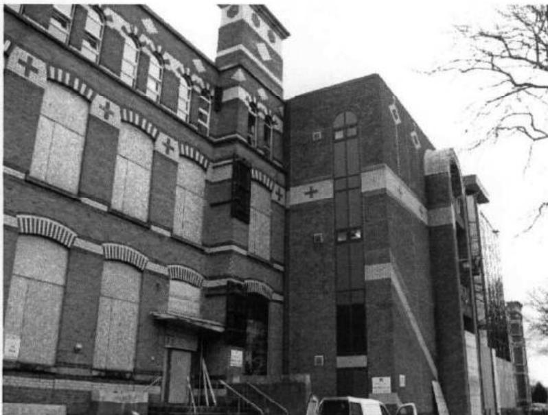
Fig. 18: 1980s addition on south-west elevation (block B)
