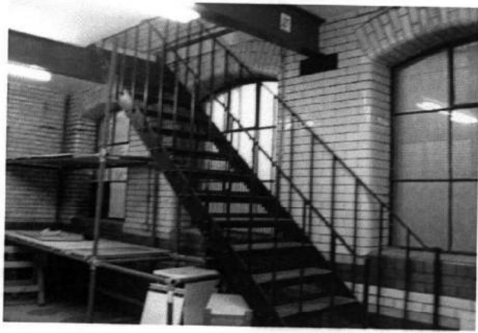
Fig.30: interior of sub station (block D)
