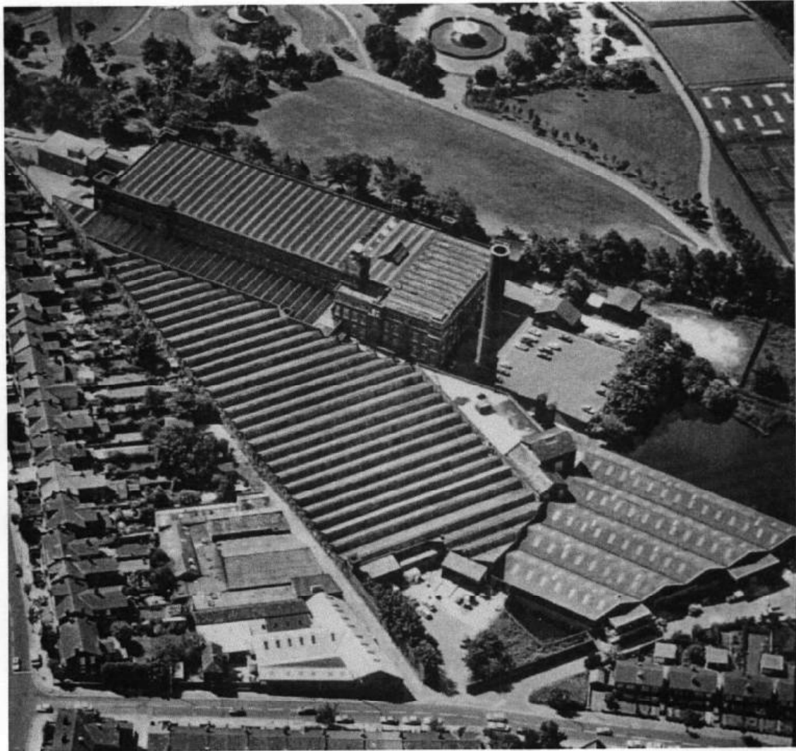
Fig.14: aerial view of the mill in the 1980s, looking south, prior to Wigan College's occupation (Greater Manchester Sites and Monuments Record ref:SF3169/20)
