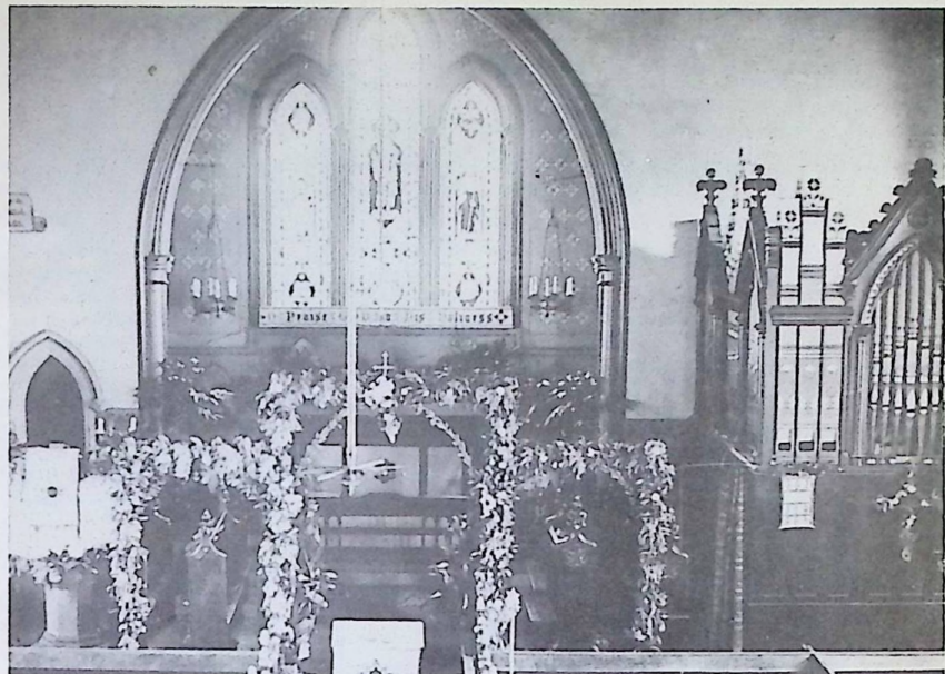
Interior of Church 1909.
