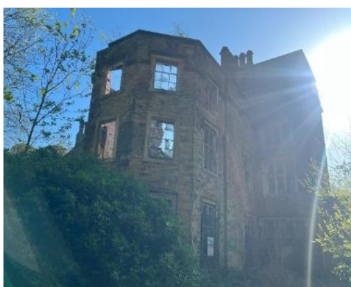
Fig 2.3 West Entrance to Winstanley Hall
