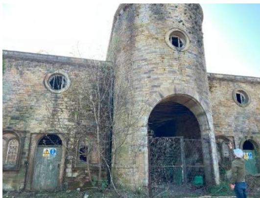
Fig 2.9 Courtyard elevation of Barn
