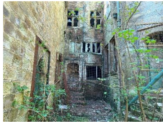
Fig 2.6 Part of the courtyard facing elevation
