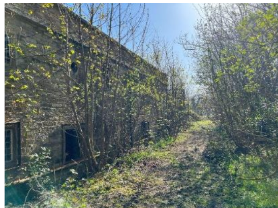
Fig 2.8 The outer facing elevation of the Coach House
