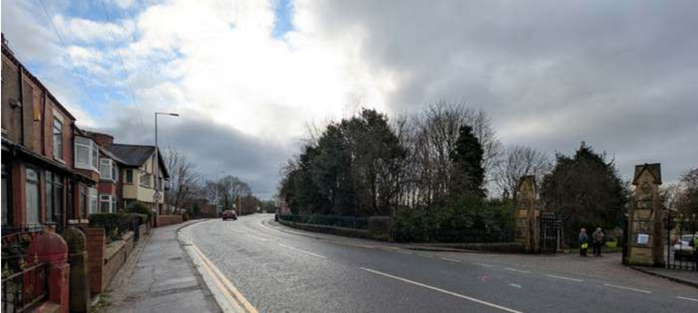
Figure 39 Main entrance approach from Warrington Road
