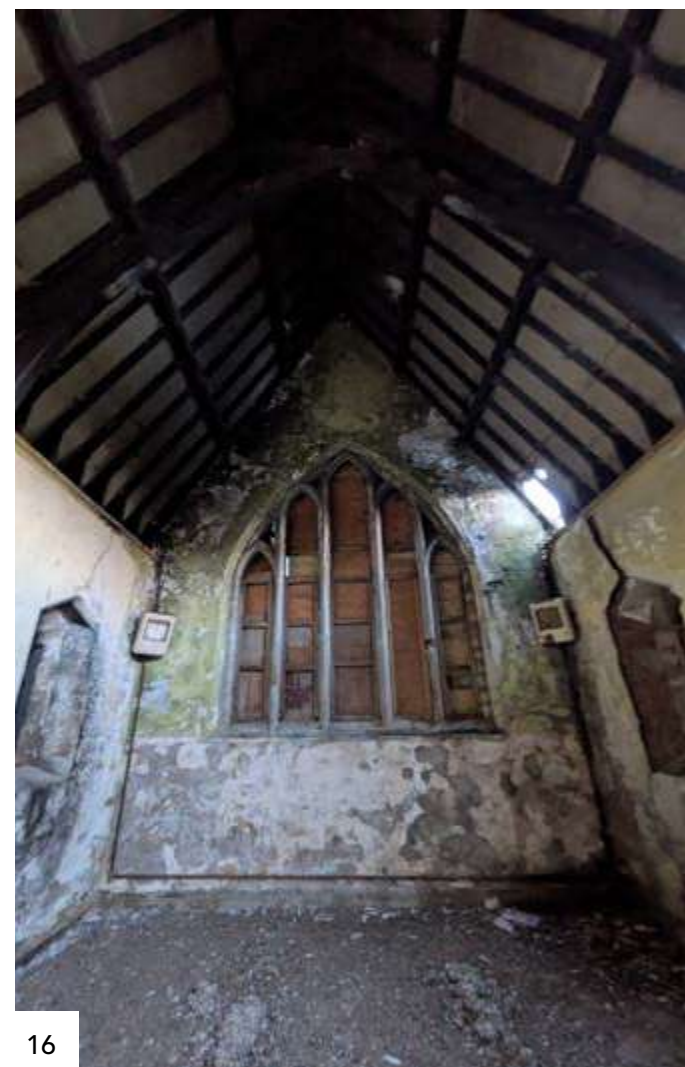
Figure 15 Evidence of original paintwork Figure 16 Gas pipework, old heaters and roof joists Figure 17 Filthy floor, exposed roof timbers Figure 18 Stepped brickwork arch detail Figure 19 Existing timber alter screen Figure 20 Missing ridge tiles, sarking board, membrane and roof timbers intact
