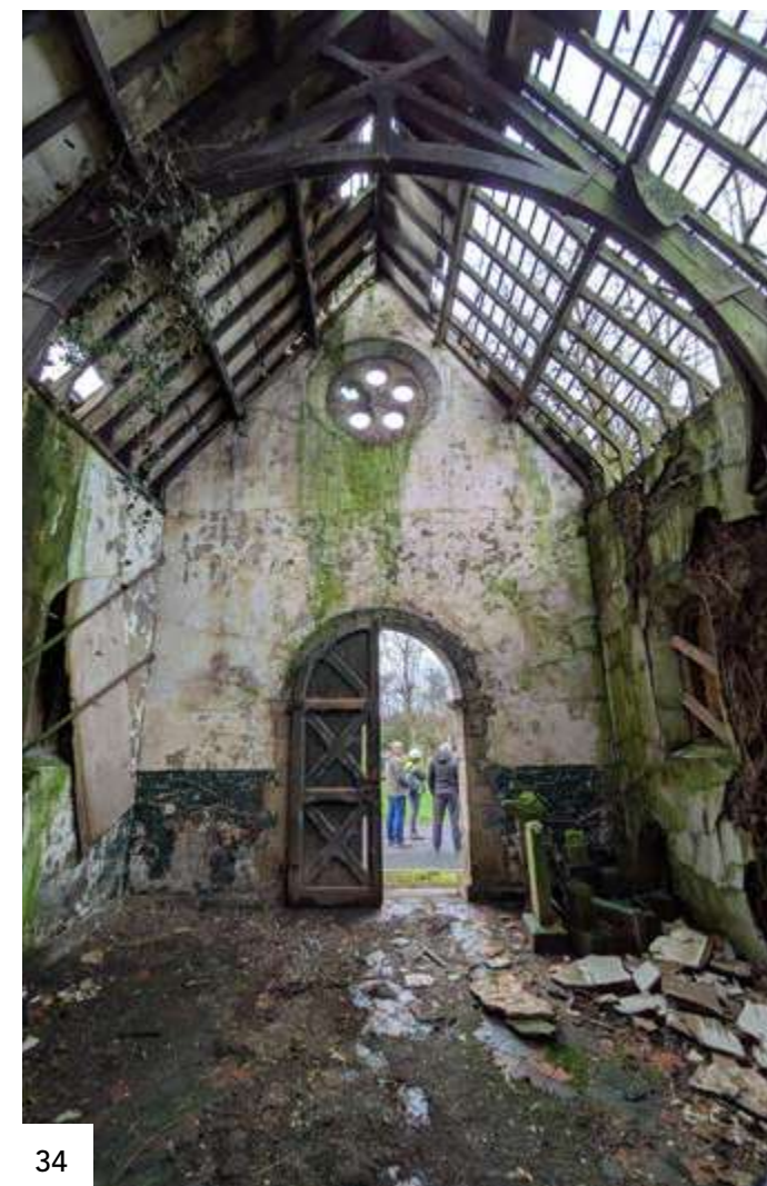
Figure 33 Roof tiles missing water ingress staining evident Figure 34 Roof covering missing Figure 35 Original paintwork evident Figure 36 Timber window frame remains, cracked plaster Figure 37 Original tiled floor Figure 38 Hole to roof-space above store
