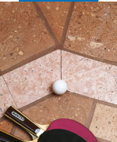
Terracotta floor polished in situ, grouted with Keracolor GG mixed with Fugolastic
