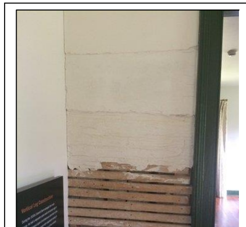
Lath and plaster demonstration in the historic home of Ulysses S Grant.
