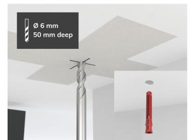
Drill the hole and install the magnet with Hilti plug and screw.
