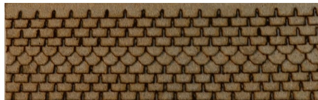
Two rows of hexagons highlight a roof edge.
