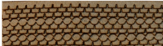
Paired rows of fish scale/reverse fish scale inserted into a standard roof.
