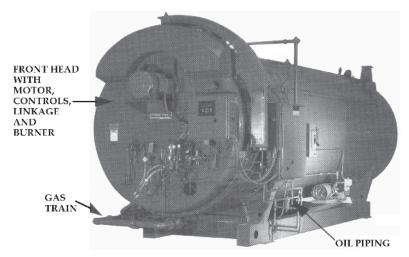
Figure 7-2. Fire Tube Boiler, Assembled
