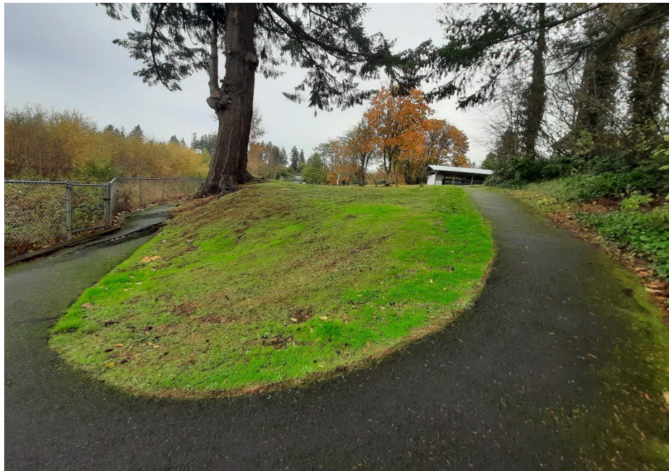
Photo 2. South of Birnie Creek, the G. Alan Johnson Waterfront Trail cuts into the natural landform and is partially built on fill. The trail segment will be replaced during the proposed project. The view is towards the northeast.
