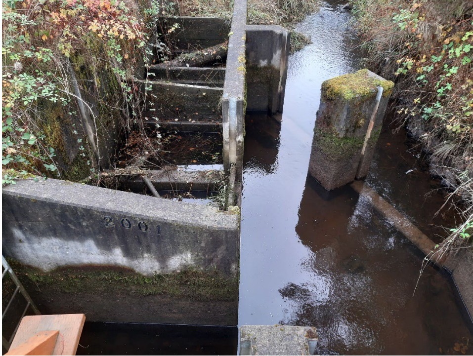
Photo 3. Birnie Creek, showing the concrete water diversion and weir constructed in 2001. The view is towards the northeast.
