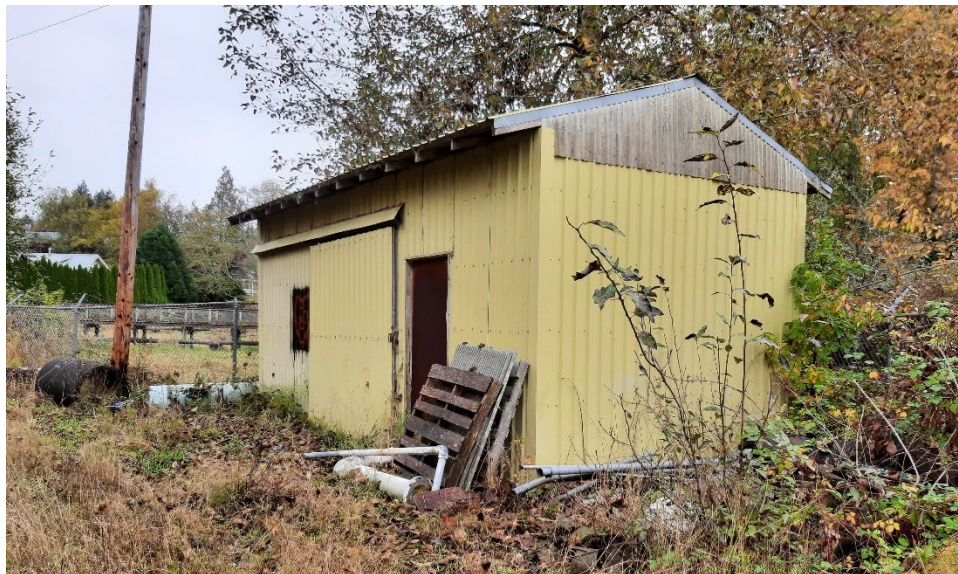
Photo 9. The post-1982 shed, located on the northern terrace of Birnie Creek, is proposed for removal. The view is towards the east.
