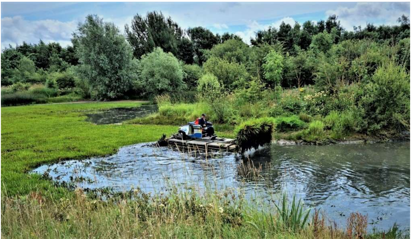
July 26 2021 Dredgers arrive and work removing an estimated 500.000 plants from the main pond
