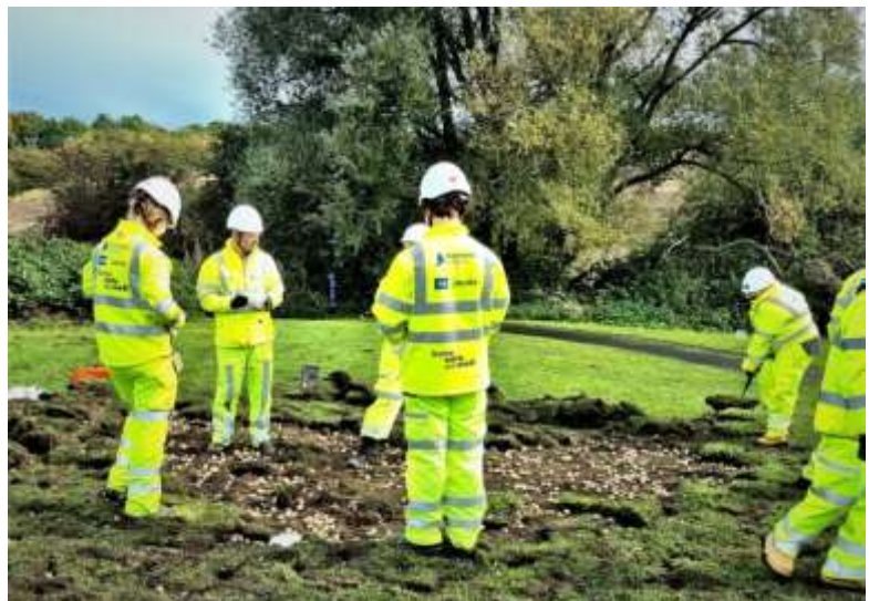
Work begins lifting the turf
