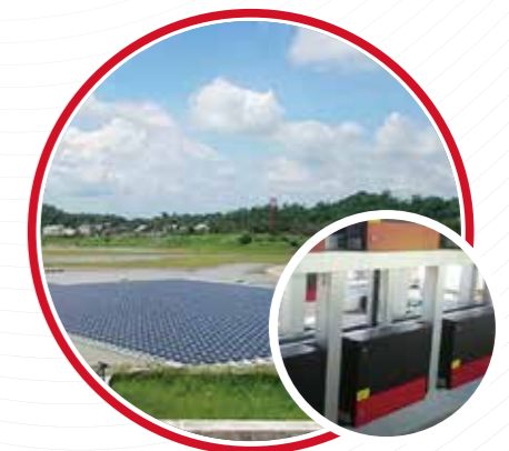
AGONG-DIAN RESERVOIR, KAOHSIUNG CITY, TAIWAN 2.3MW
