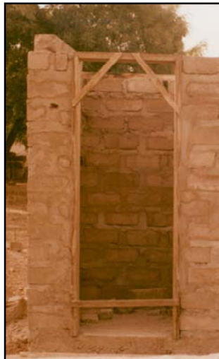
The toilets under construction
