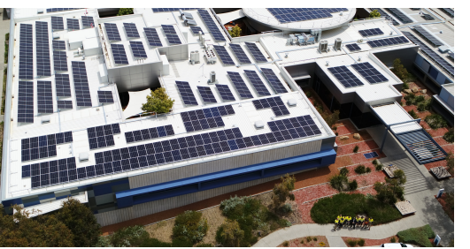
Project 310kW solar panel installation Client Water Corporation Scope Installation of 688 solar panels (310kW) Value $1.3M
