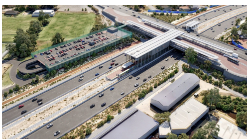
Project Melconnx Ellenbrook to Morley Line Client Laing O'Rourke Scope Supply and installation of site services across five sites. Value $320K
