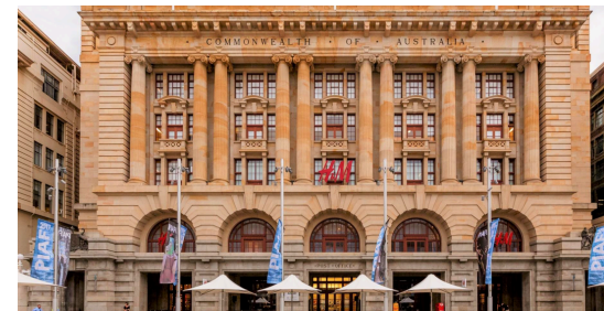
Project Multiple H & M Fashion Outlet Stores Client Swan Group & Valmont Scope Supply & installation electrical, lighting & comms services Value $2.2M
