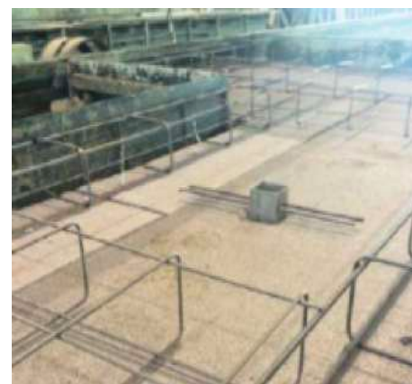
Isolante posato Insulation installed
