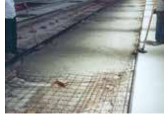
Concrete bed preparation
