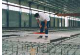
Checking the level of the rails
