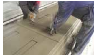
Operators working on the fresh concrete marked out by the plotter
