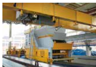
Casting machine being lifted by the concrete distributor
