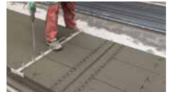
Operators working on the fresh concrete marked out by the plotter
