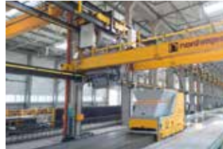
Fly bucket filling the concrete distributor
