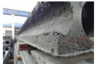
Hollow core slabs longitudinally cut by fresh concrete saw
