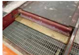
Safety grate for debris conveyor chain
