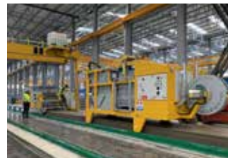
Concrete aspirator working behind the casting machine
