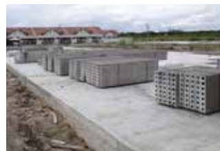
Partition wall panels on-site
