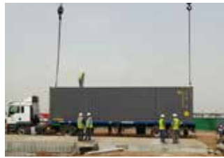
Installation of the heating plant container
