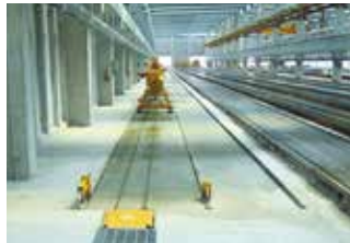
Concrete element transport line
