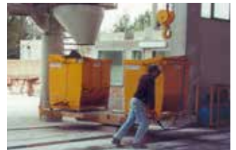
Bucket being loaded under the mixer
