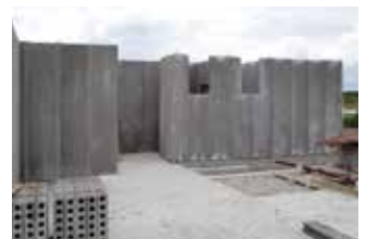
Erected partition wall panels
