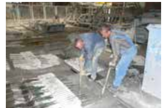
Water being collected manually without the debris conveyor chain
