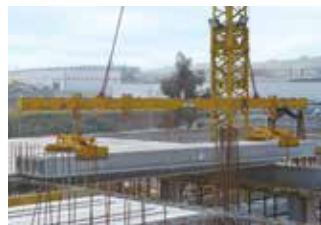
Mechanical fixed lifting beam for hollow core slabs
