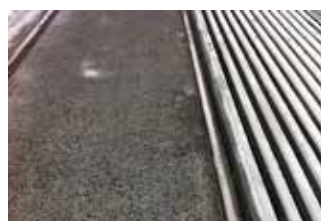
Concrete bed recently polished
