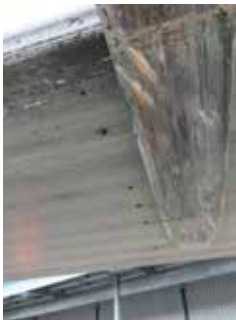
Hollow core slabs with holes
