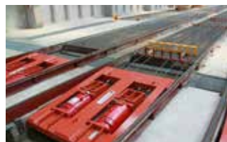
The detensioning cylinders installed in the reaction beams
