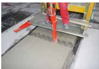
Concrete being removed at the cutting point to expose the wires
