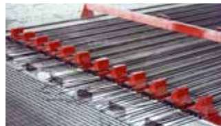
Reaction beam with reaction spacer incorporated
