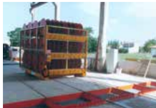
Coil holder trolley during the laying of the steel wires
