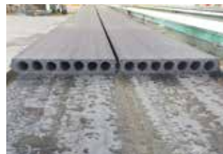
Production of 2x600 mm wide wall panels
