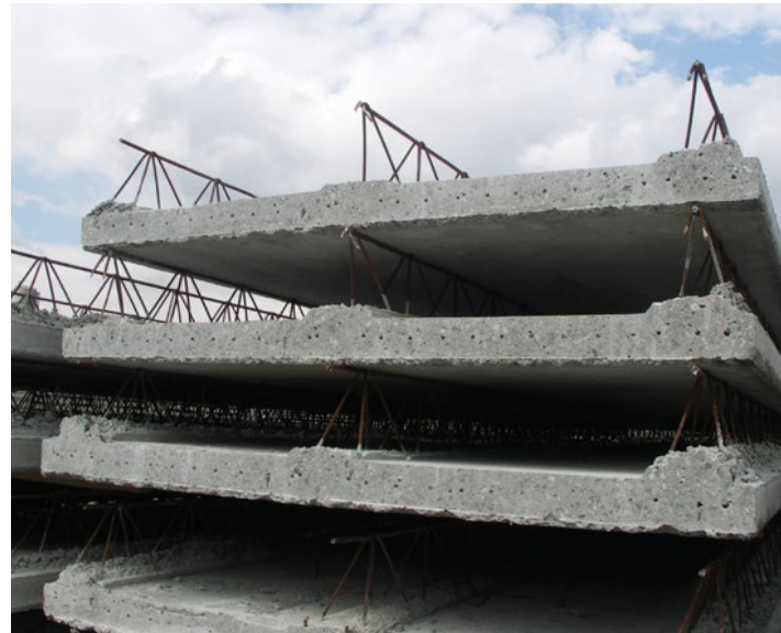
SLABS WITH LATTICE RIBS
