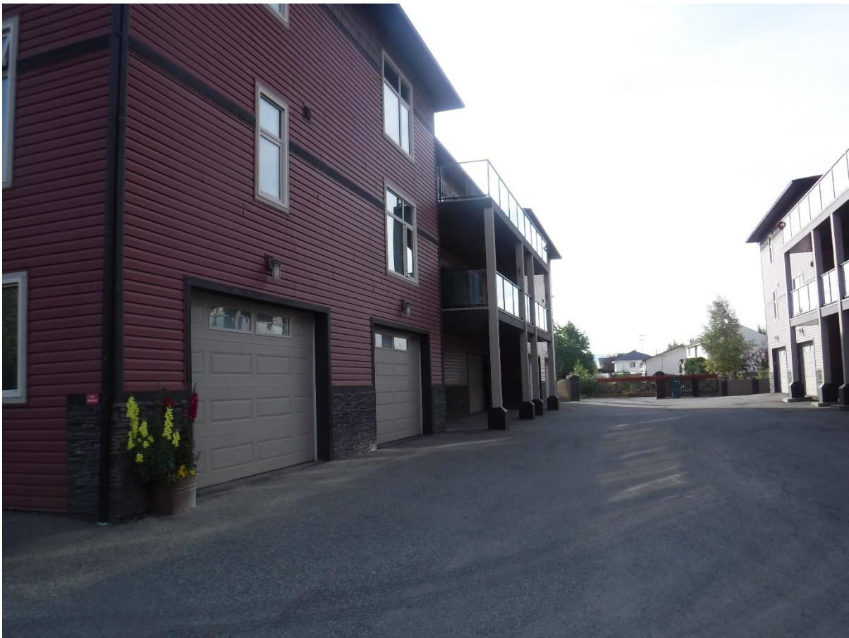
The view of the parking lot looking towards the front gate. Building A is on the left. No cracks.
