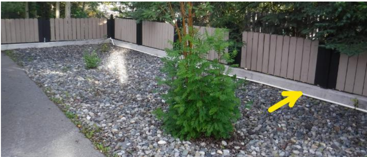
The yellow arrow points to the PVC drainage pipe that carries excess water off the property.
