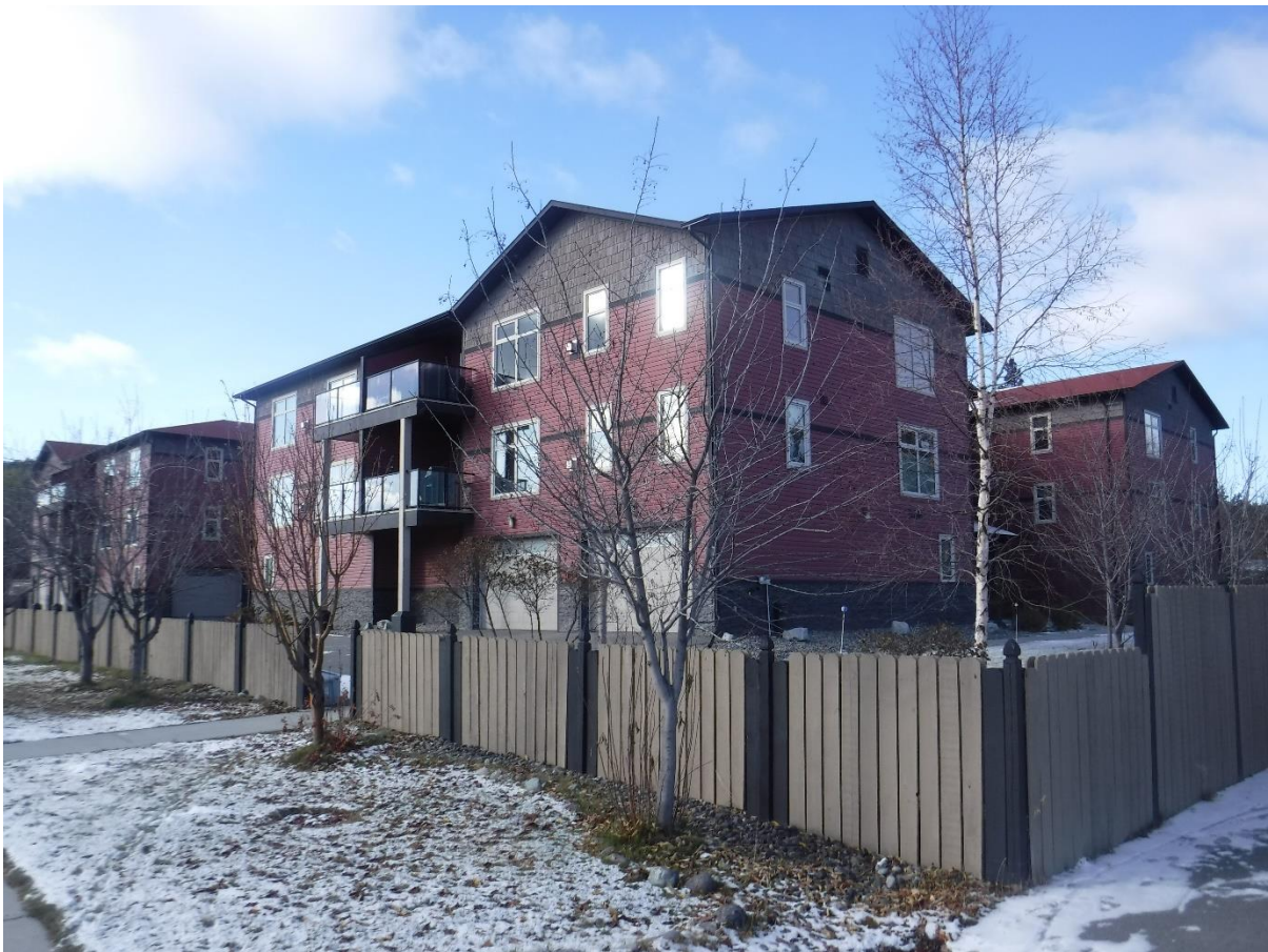
A good view of the windows from the south-east corner of the complex.
