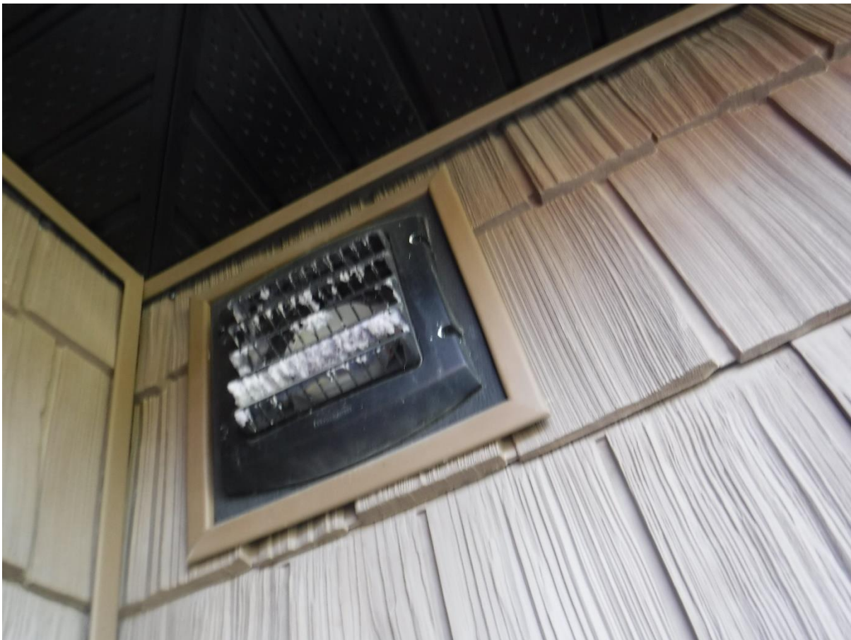
A vent on an exterior wall. The cladding is vinyl.
