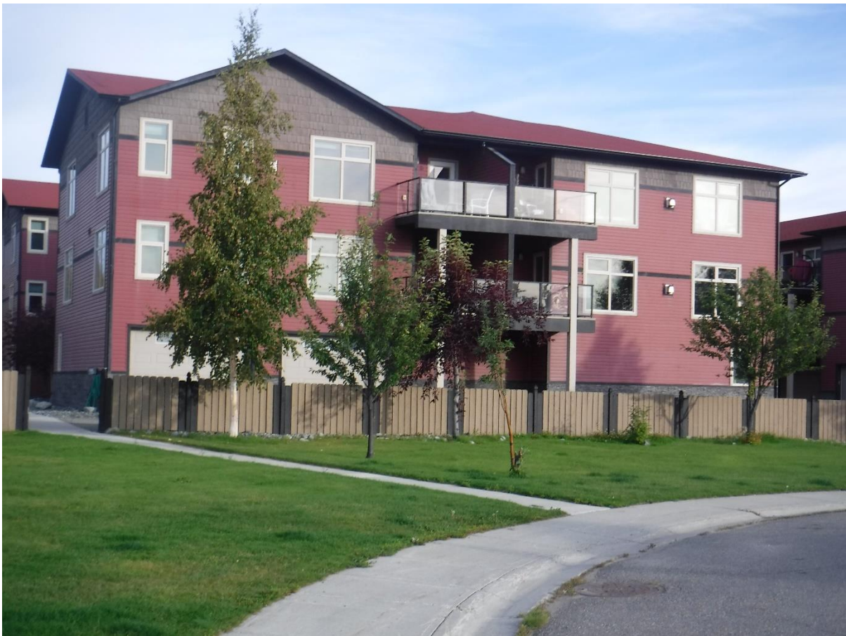
The front fence looks great.
