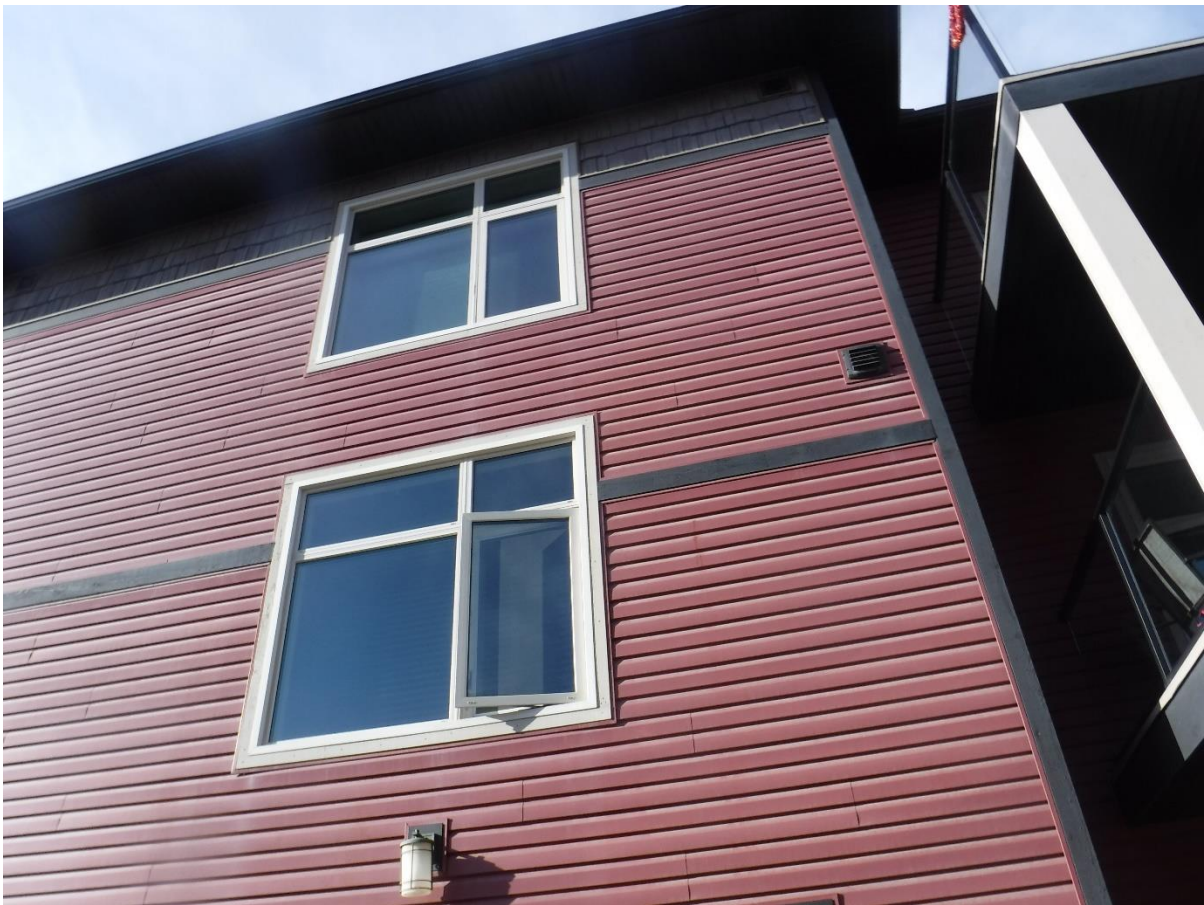
Two larger casement windows.
