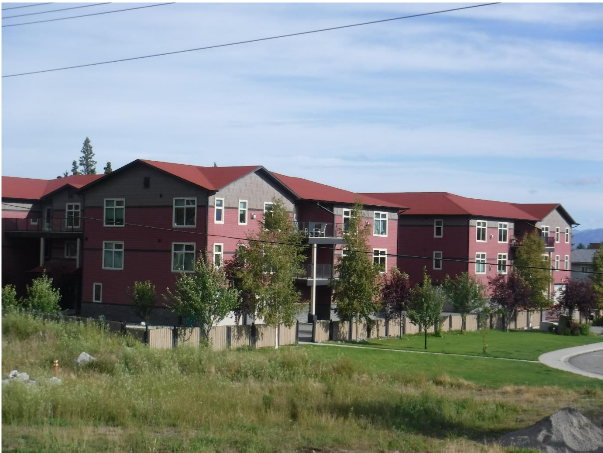
View of the Lansing Point condo complex from the Alaska Highway. The roof angles are more visible than from an on-site vantage point.
