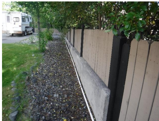
The concrete wall on the eastern property line.
