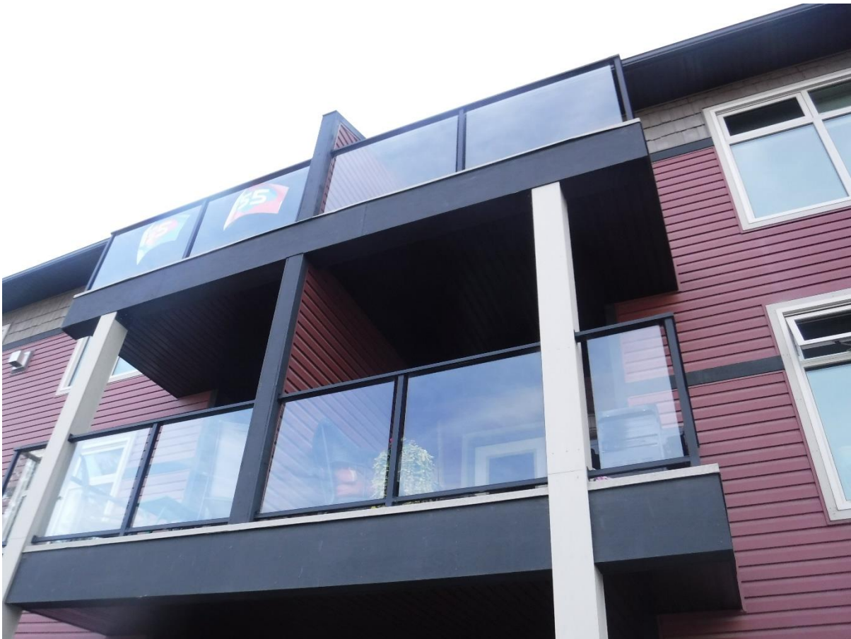
Looking up at the balconies for 4 units.
