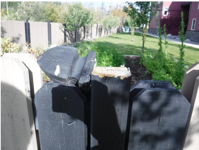
This ornamental top of the fence post has broken off.
