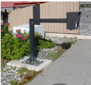
Gate control interface.
