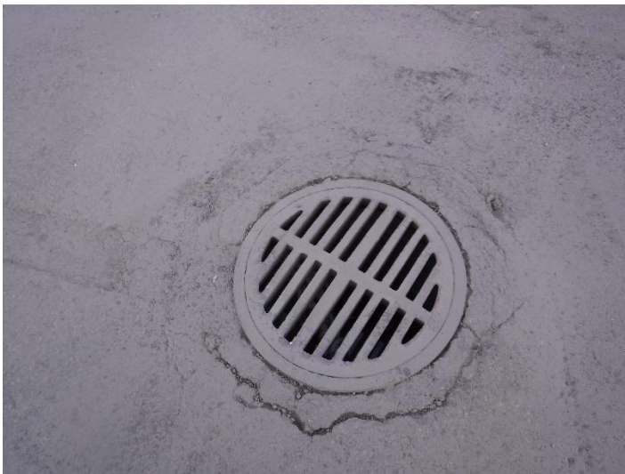
A manhole for one of the two catch basins located in the parking lot.
