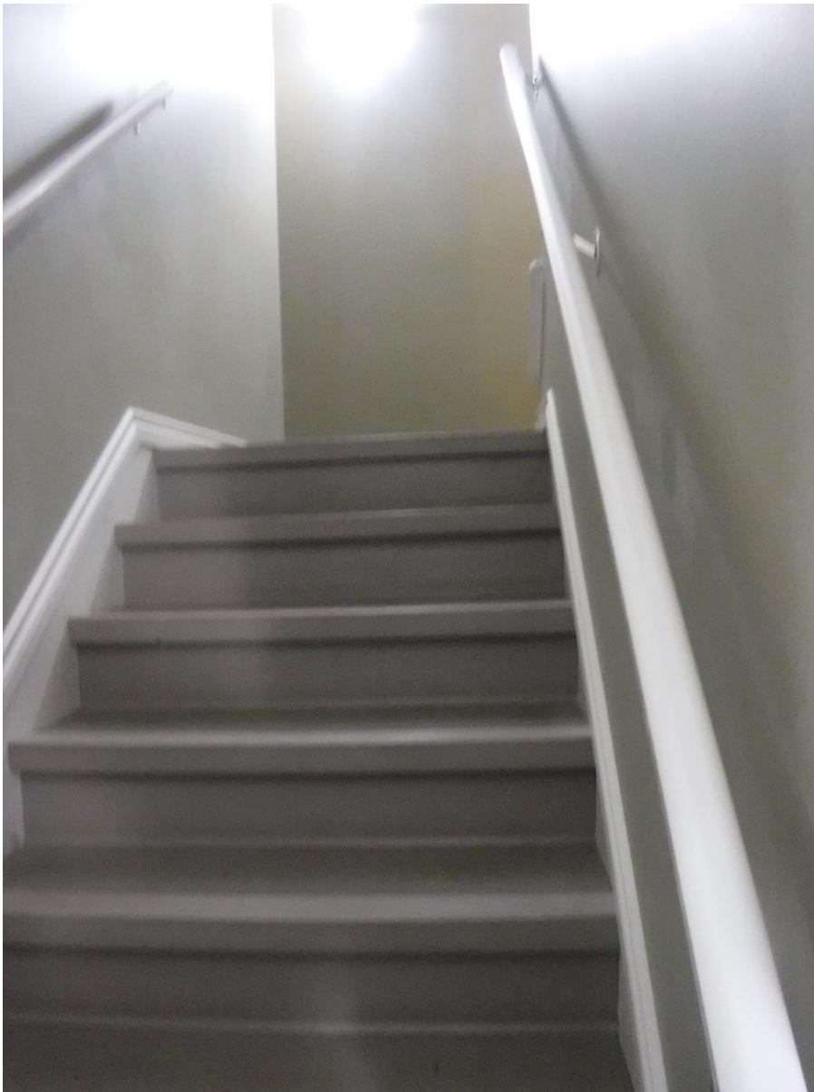
The stairwells between floors are nicely finished with paint and trim.
