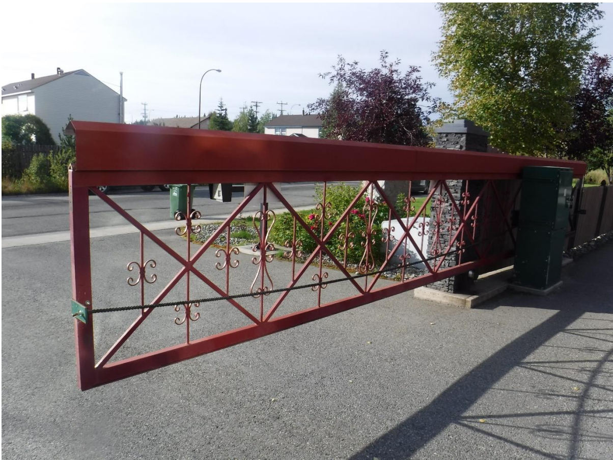
The automated front gate.
