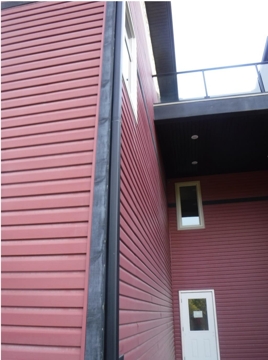
View of a corner. Vinyl siding and wood trim.
