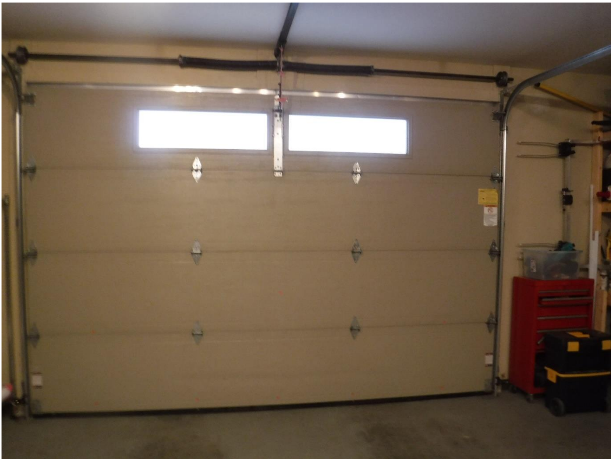
Garage door – view from the inside.
