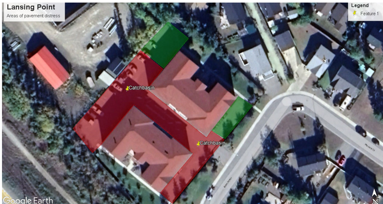
Figure 2: Google Earth image showing pavement cracking areas in red and areas of little to no cracking in green
