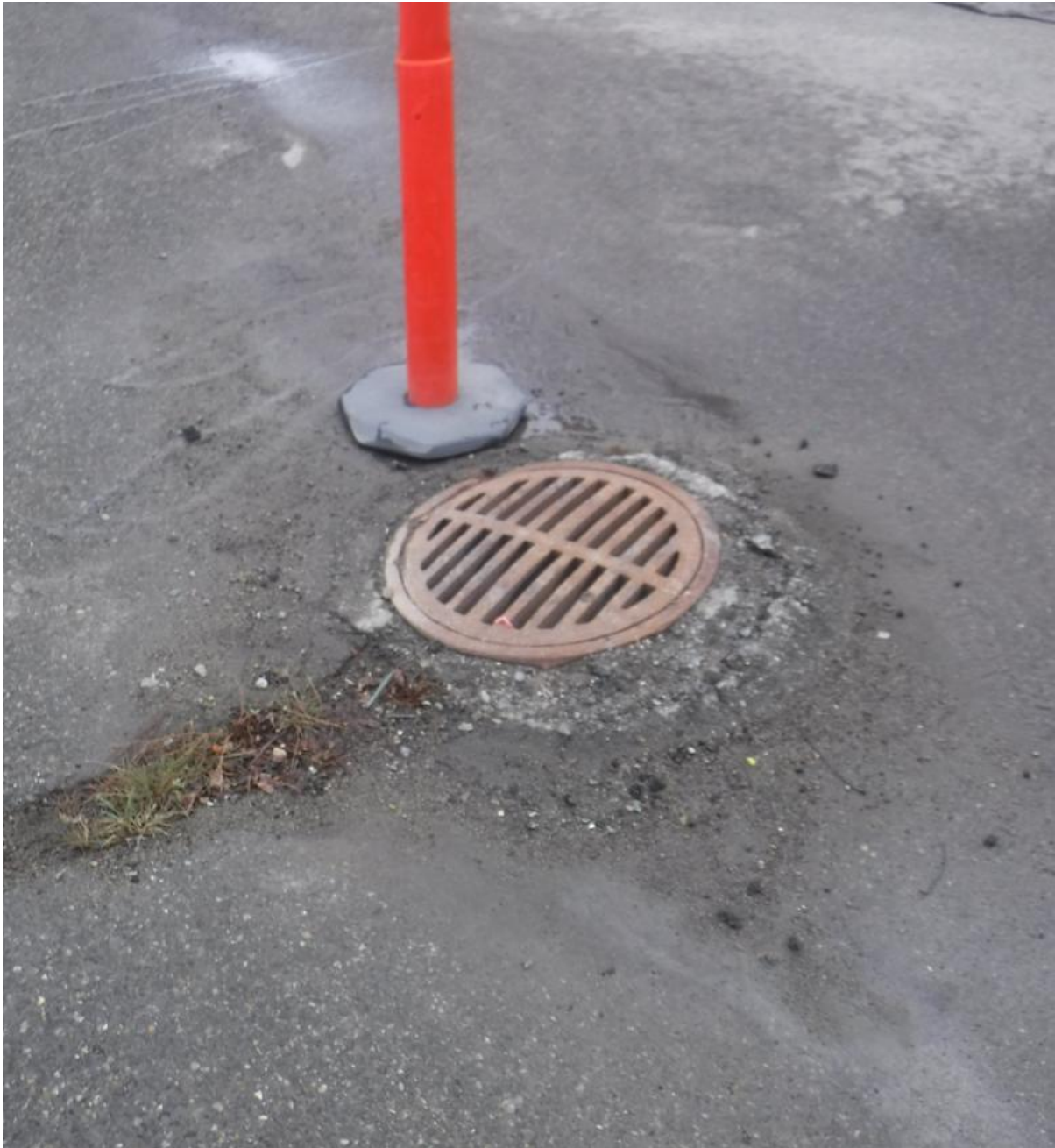
Subsidence and asphalt damage around a catch basin.
