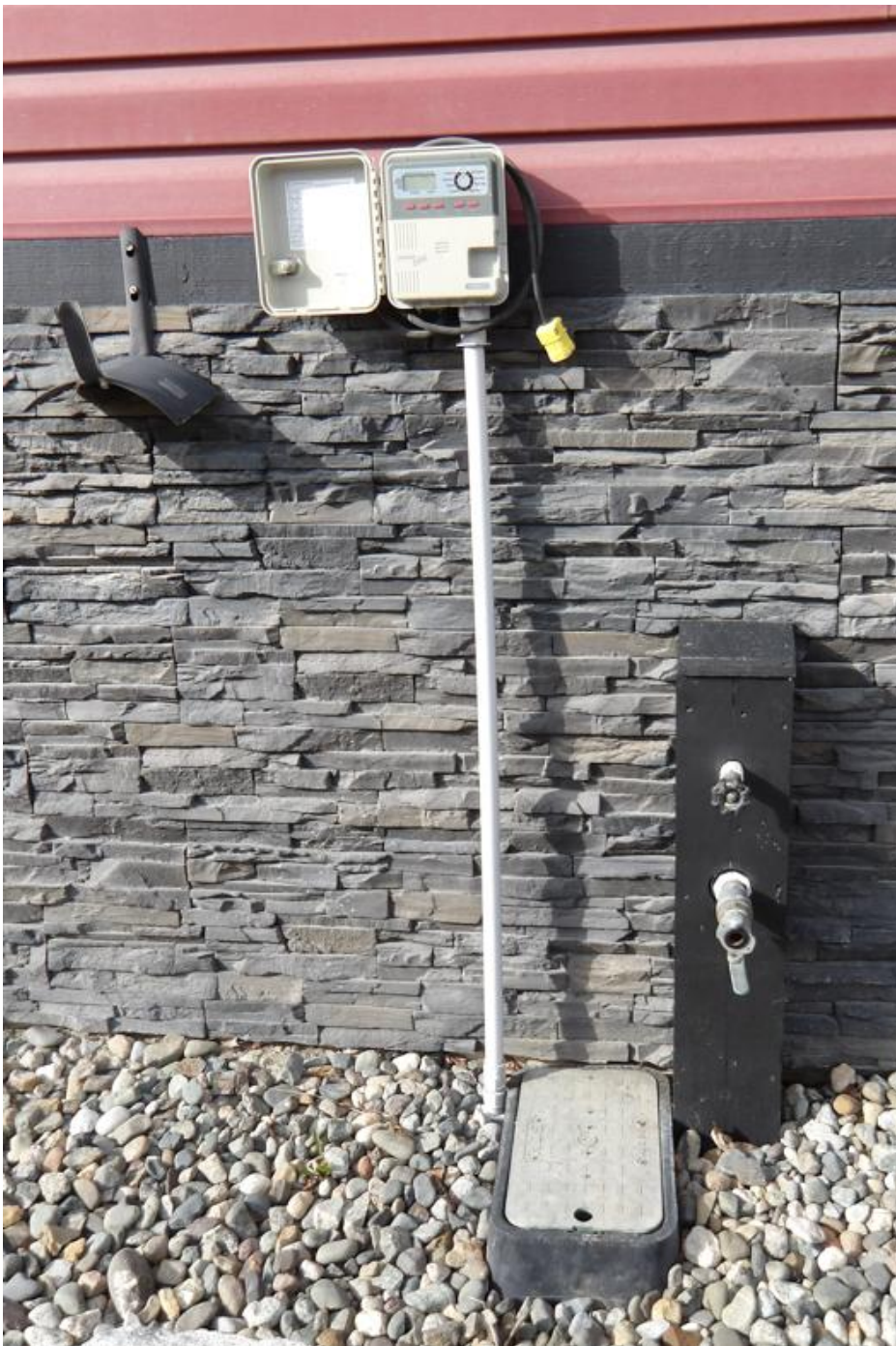
The control panel for the irrigation system.
