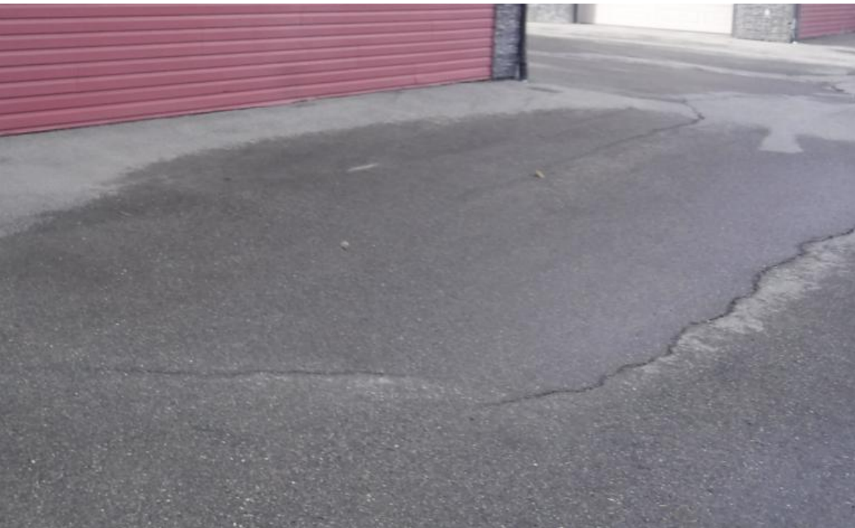
Long curved crack.
