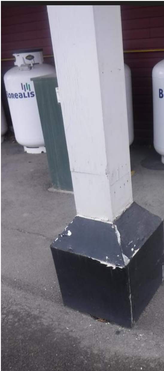
A support column wrap. The base wraps of balconies structural supports will be repaired in 2025.
