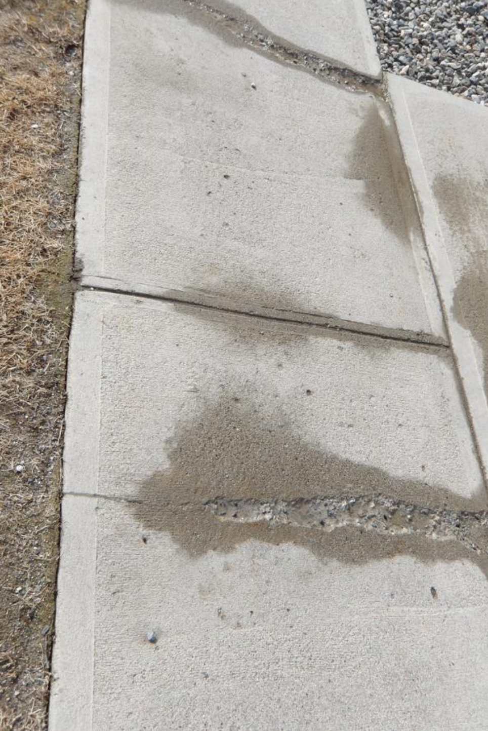
Large cracks/erosion in these sidewalk sections.
