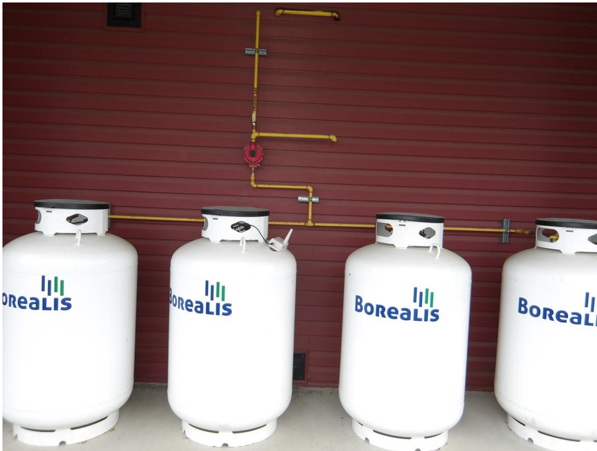
The yellow pipes connect the propane tanks to the units in the building.
