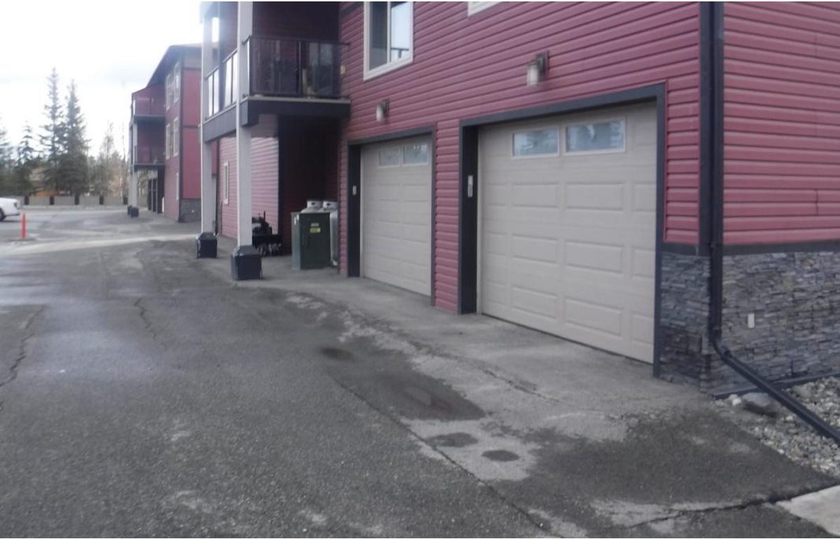
North parking lot. Numerous cracks. These can be inexpensively filled.
