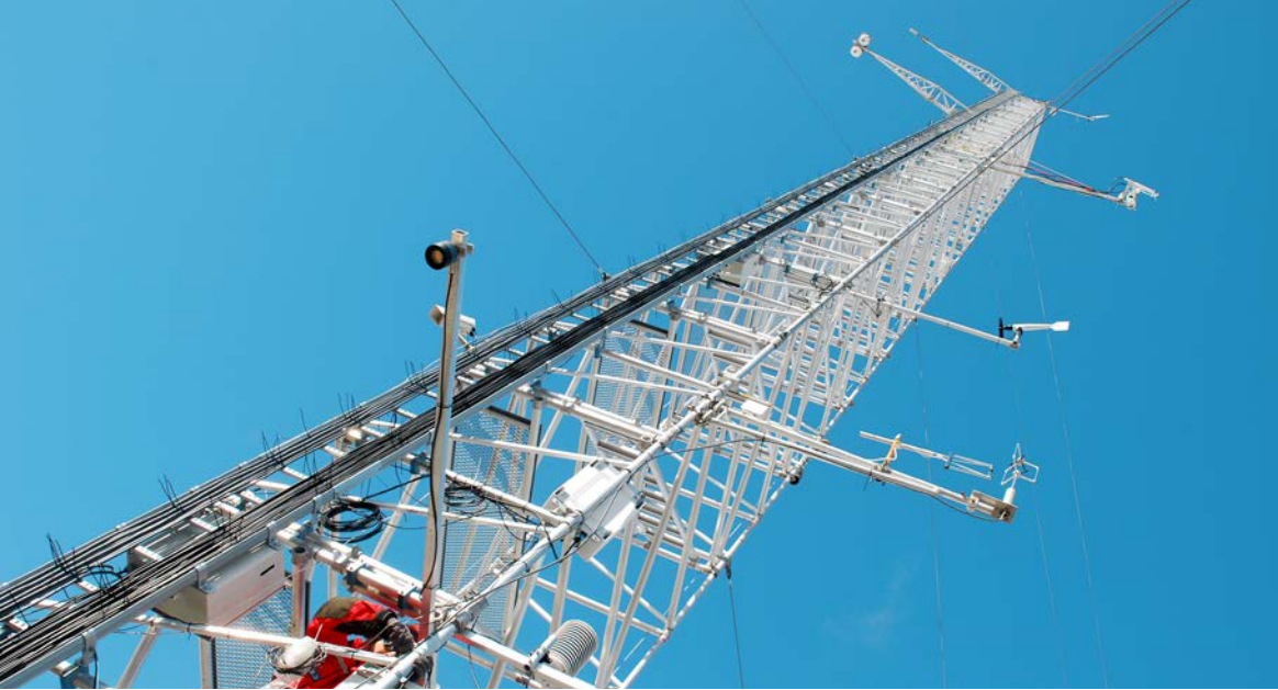
← The Amundsen-Nobile Climate Change Tower during maintenance. © Fabio Giardi
