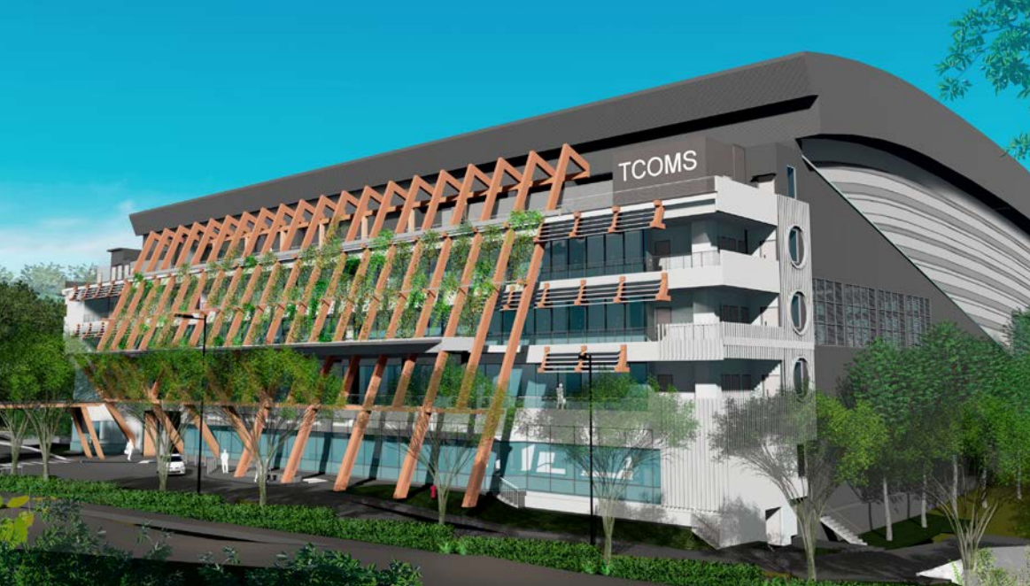
← Artist's impression of the Technology Centre for Offshore and Marine Singapore (TCOMS) facility. © National University of Singapore
