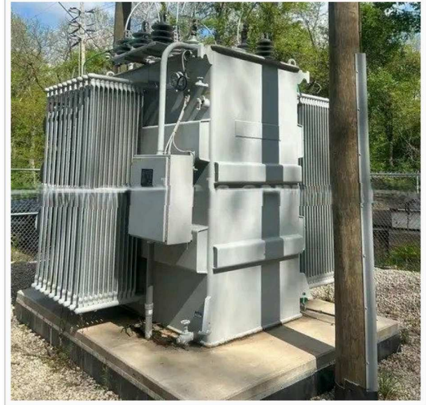
Reconditioned 7,500 KVA Sunbelt substation transformer
