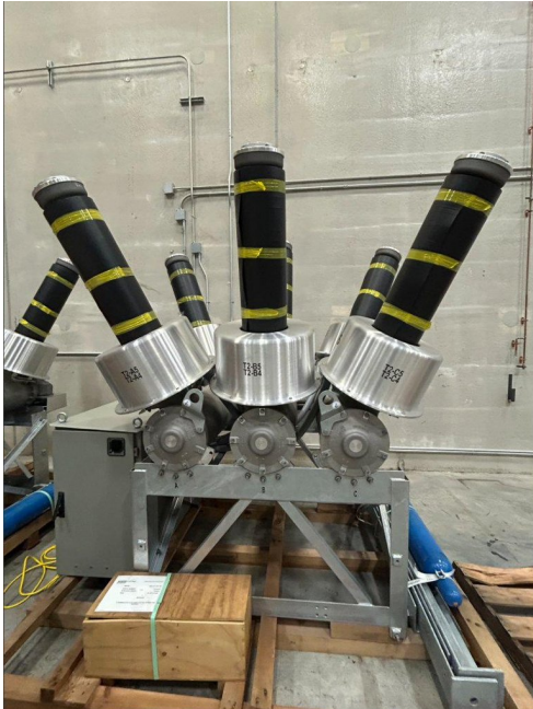
Front view: three SF6 bushings and dead tank
